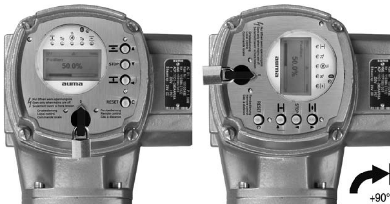
Figure 9: Mounting positions C-2 and D-2
