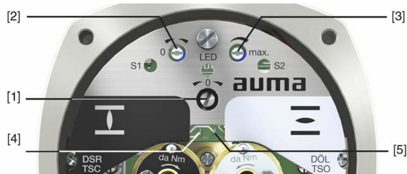
Figure 69: View on control unit when switch compartment is open
