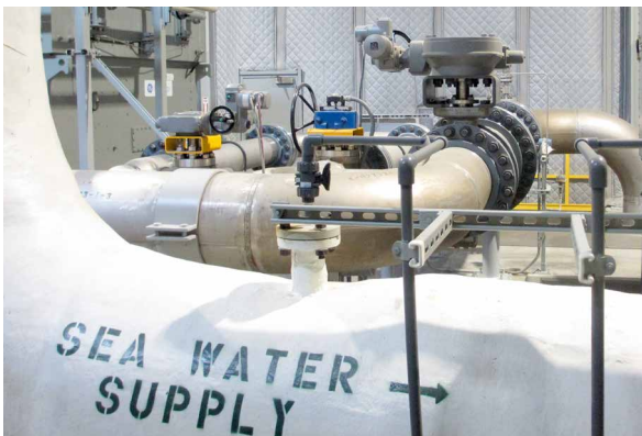
In places where high-performance pumps cause strong vibration, the actuator controls are mounted separately from the actuators.
