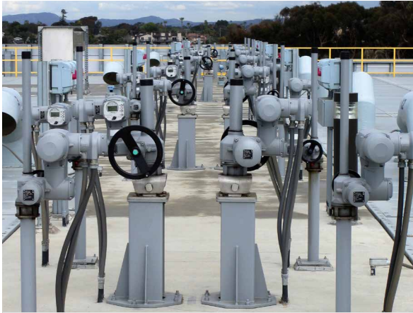
No trace of corrosion: Thanks to their TÜV-certified corrosion protection AUMA actuators withstand the salty sea air at Carlsbad.
