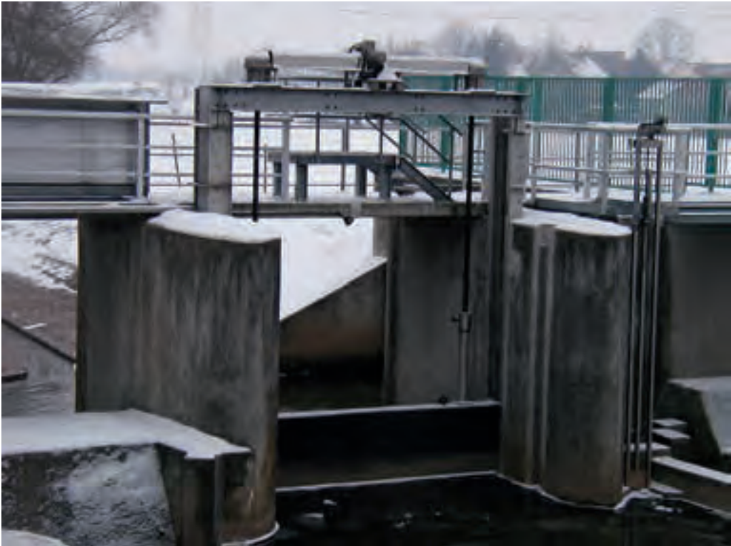
Figure 2.081: Non-rising spindle at sluice gate with 3-side seal
