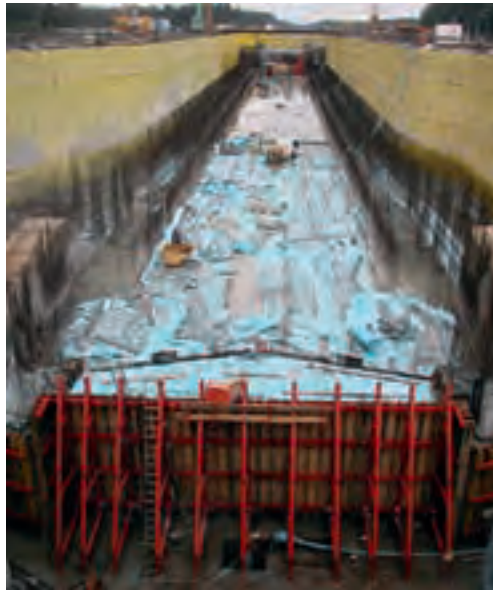
Figure 8.02: Lock building site. The concrete work is being prepared
