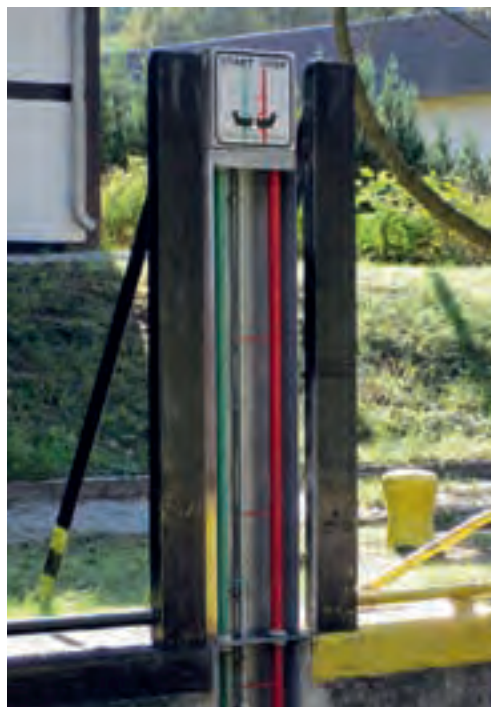
Figure 3.33: Automatically operated lock: “Turn the green lever for locking!”
