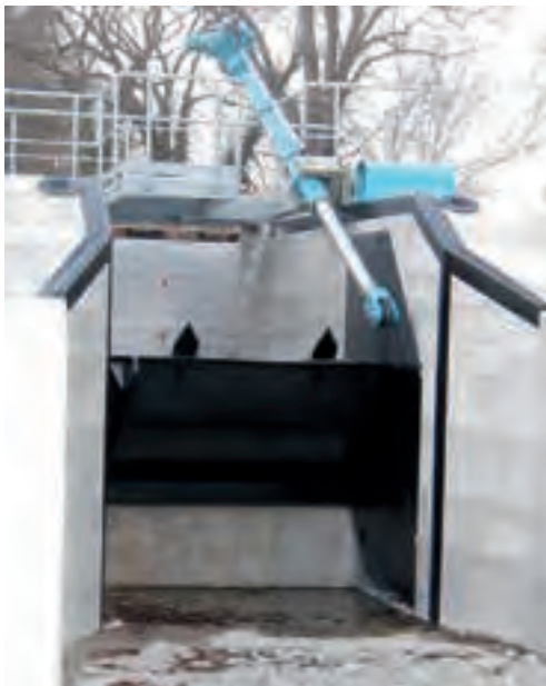
Figure 2.141: Shutter with actuator and gimbal mounted lifting cylinder
