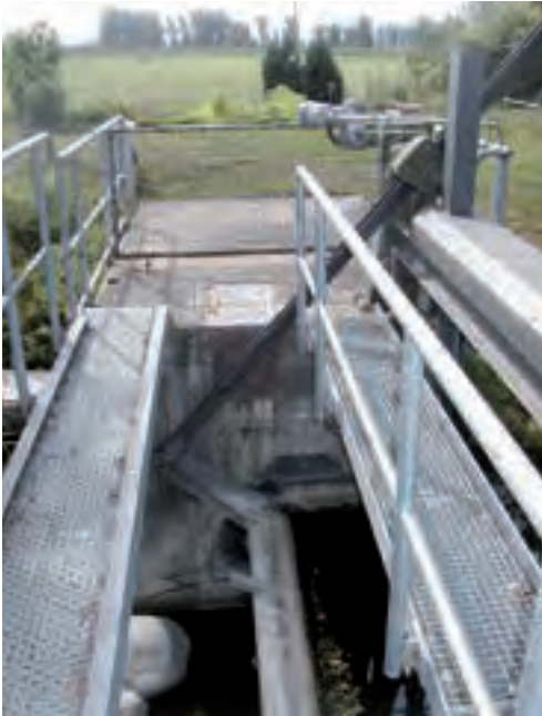
Figure 1.14: Shutter weir
