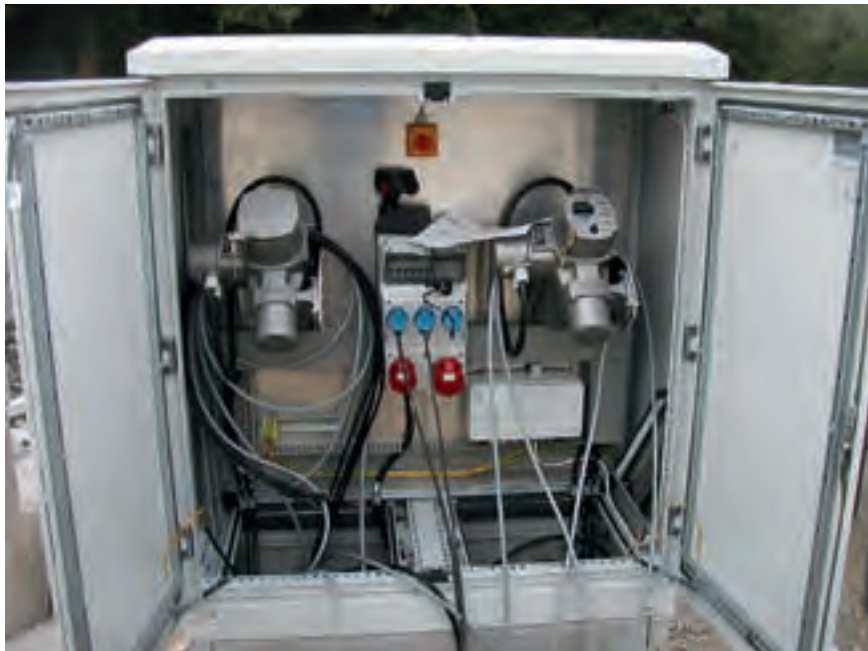
Figure 8.06: Connecting AUMATIC actuator controls
