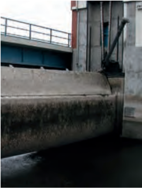
Figure 2.150: Sluice gate weir lifted with chain hoist. Fish-belly flap gate was straightened up thanks to electrical lifting cylinders
