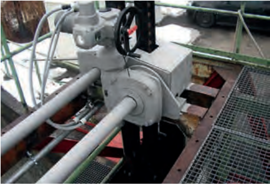
Figure 2.103: One worm gearbox operates two pinions
