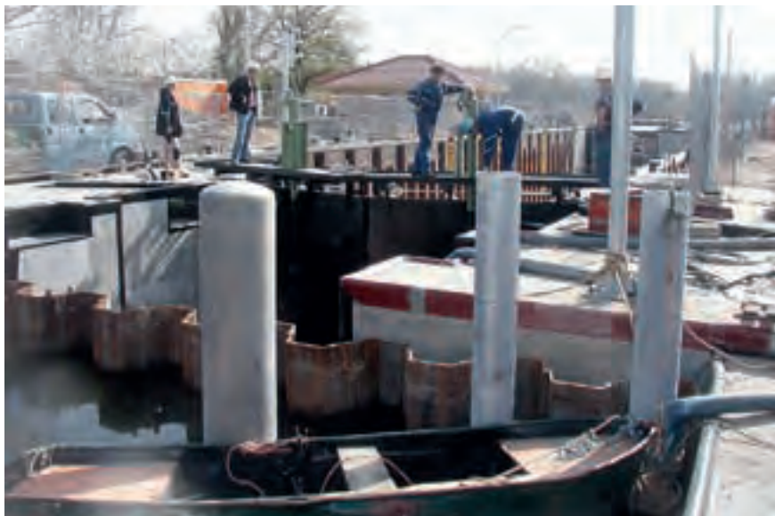
Figure 8.05: Last actions for actuator installation
