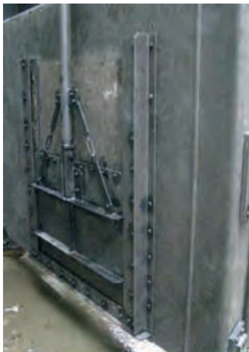
Figure 3.10: Adjustable sliding gate within a mitre gate, headwater side
