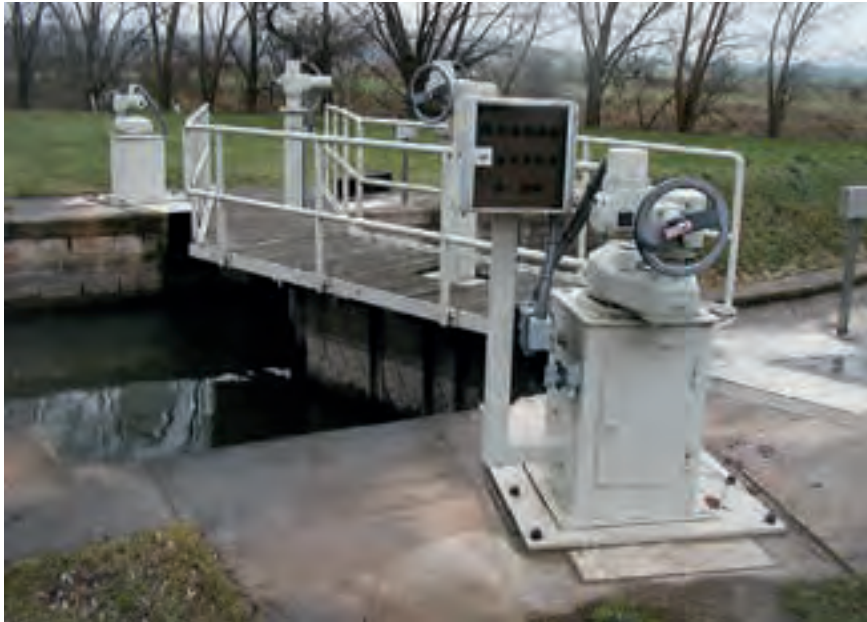
Figure 4.06: NORM actuators with common local controls at lower lock gate
