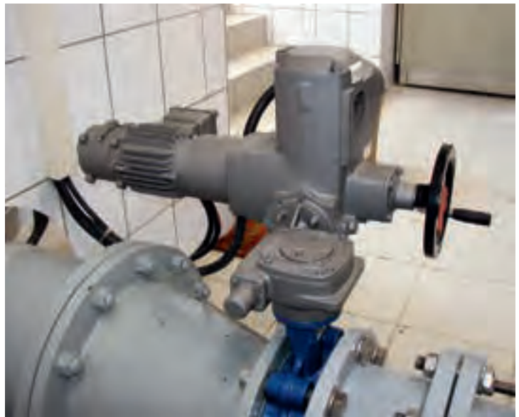
Figure 4.42: Actuator with emergency power supply 24 V DC
