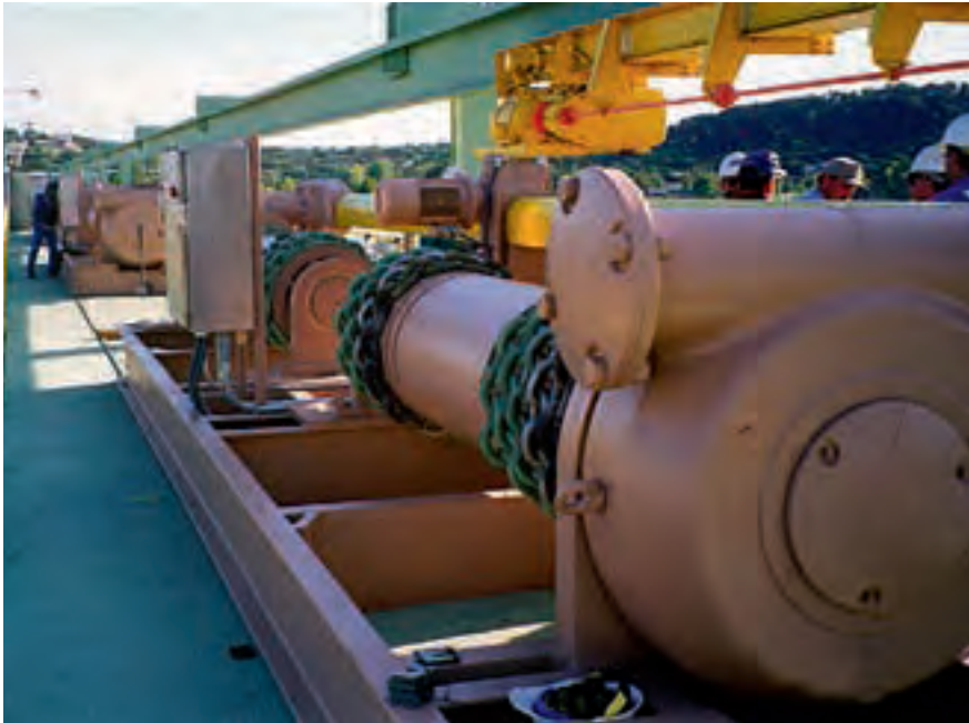
Figure 2.117: Hoist unit with link chains, in front GS 400 worm gearbox
