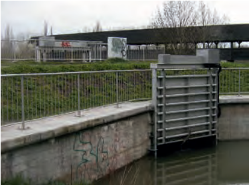
Figure 6.02: Completely housed actuator – bevel gearbox set-up
