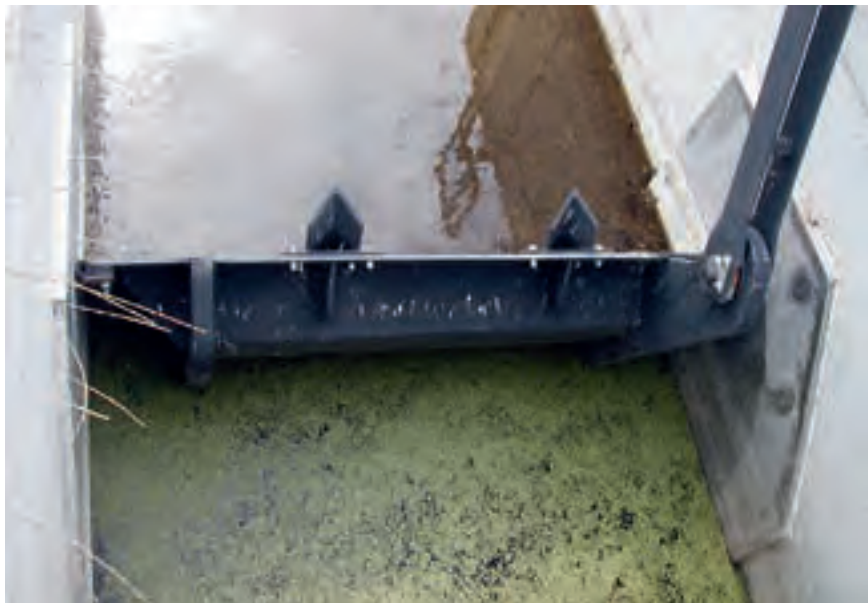
Figure 2.137: Shutter with trapezoidal profile reinforcement, tailwater
