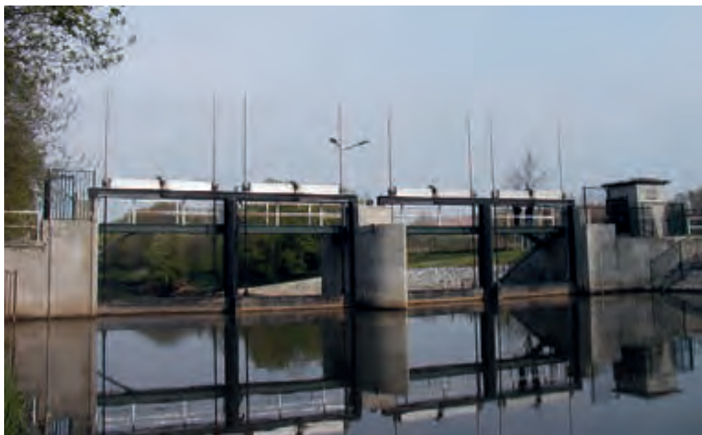
Figure 9.04: New: Weir with electro-mechanical operation via Profibus
