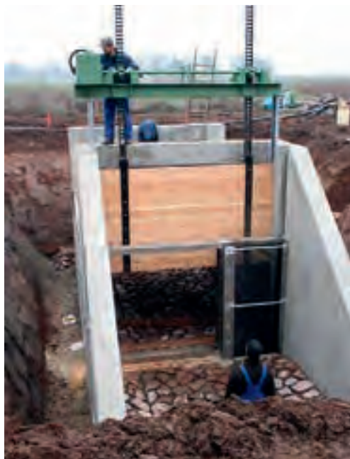
Figure 2.101: Side mount of worm gearbox with handwheel. Pinion shaft diagonally to the flow direction
