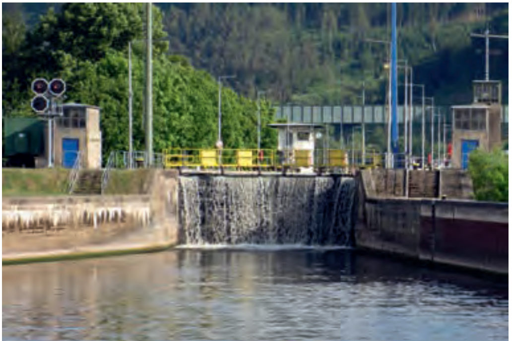
Figure 3.08: Water overflows the tailwater side due to premature opening of the headwater side
