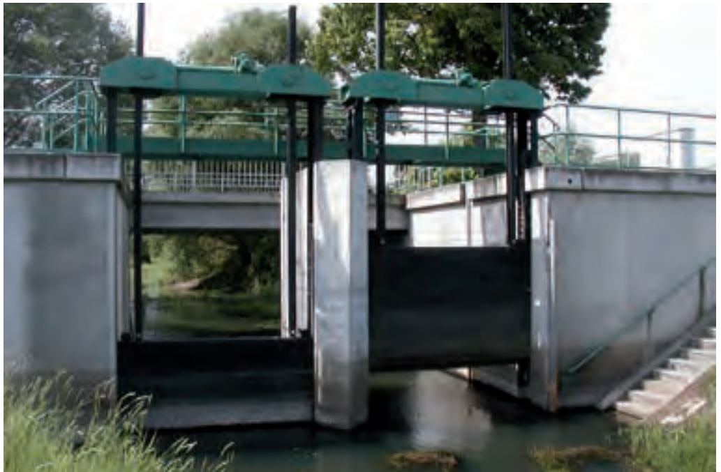
Figure 2.004: Sluice gate weirs with two lantern gears
