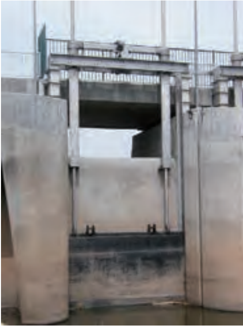
Figure 2.005: By-pass seal sluice gate in front of a baffle
