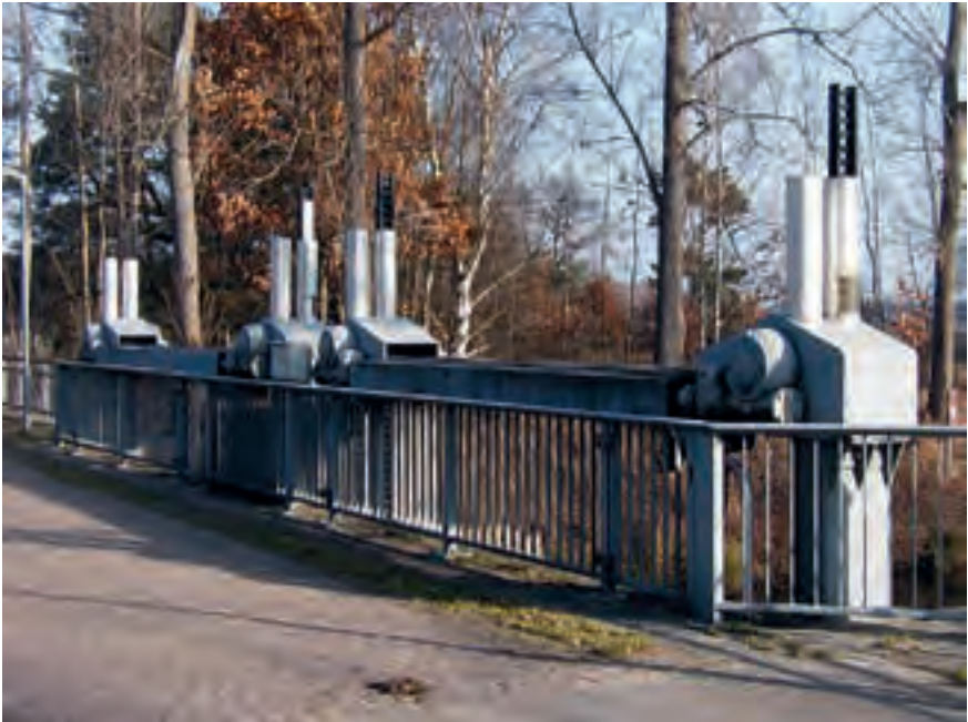
Figure 5.02: Weir with lantern gear protection tubes
