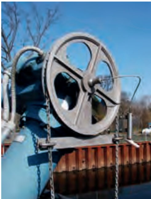
Figure 2.070: Manual operation via Bowden cable and link chain
