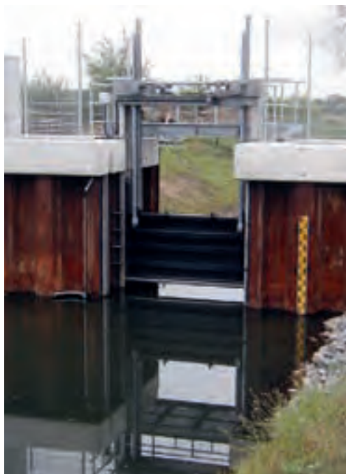
Figure 2.061: Visualisation by means of a level rod at a double gate weir
