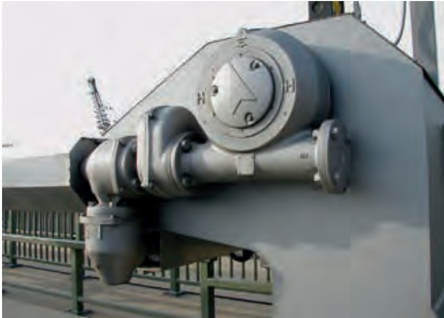
Figure 2.133: Tailwater side lower shaft cross-over of actuator to the headwater mounted gearboxes
