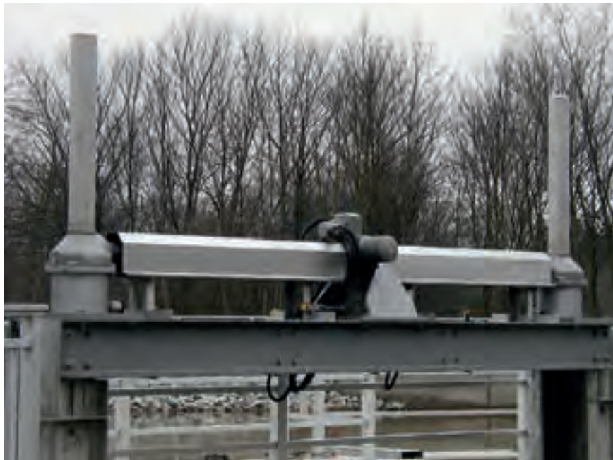
Figure 5.05: Weir with covered connecting shafts
