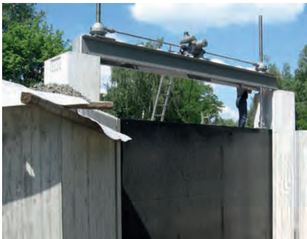
Figure 2.074: Actuator simultaneously generates clockwise and counterclockwise revolution at gearbox inputs and outputs
