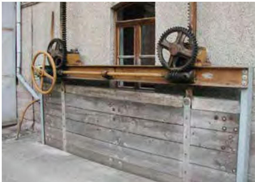
Figure 1: Shutter weir with open mechanics
