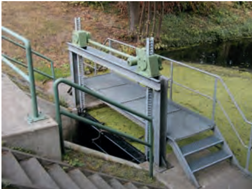
Figure 9.07: New: Sluice weir with electro-mechanically operated lantern gears
