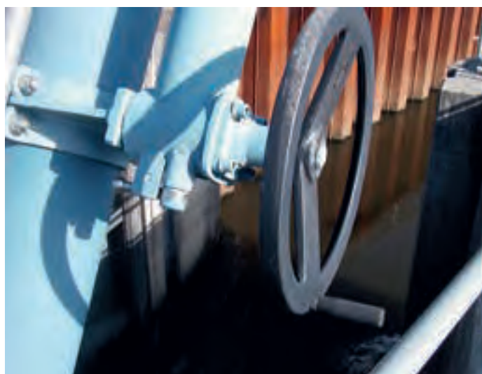
Figure 2.072: Motor/manual handwheel activation
