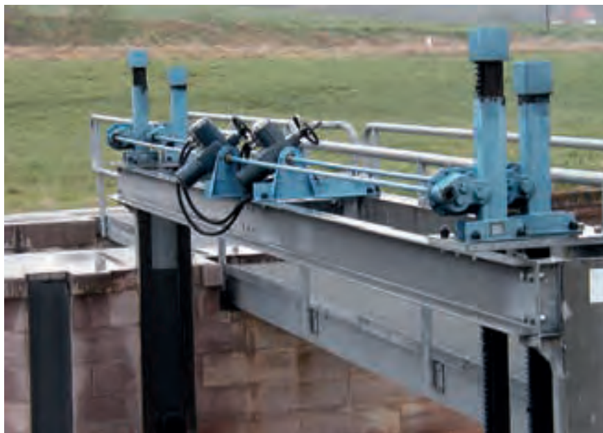
Figure 2.090: Toothed racks are operated sideways by the centre mounted actuators via pinions
