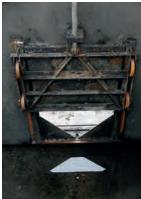
Figure 3.11: Wedge roller gate within a mitre gate, headwater side
