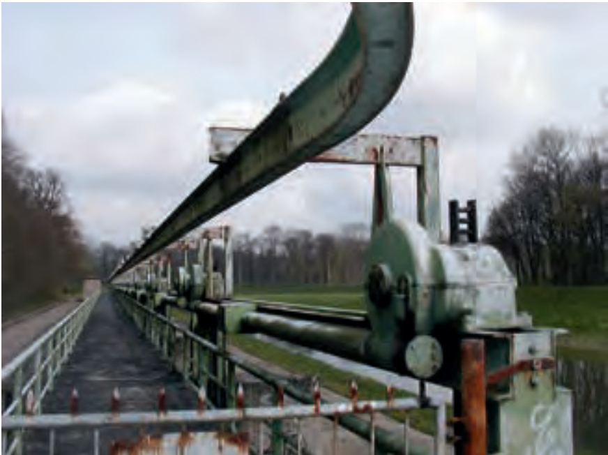
Figure 4.40: A rail actuator operates 16 sluice gates
