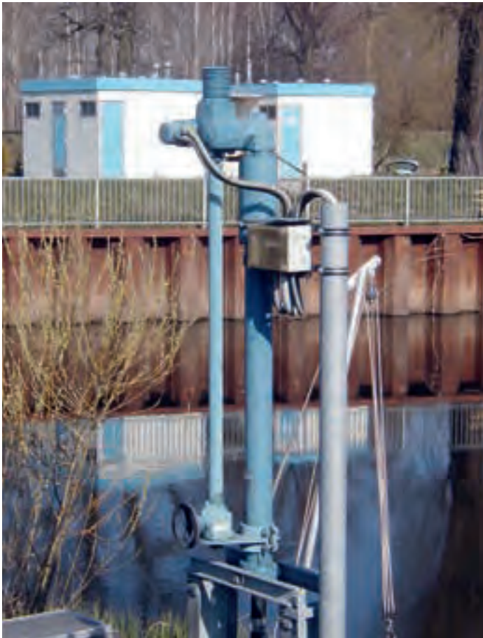
Figure 2.073: Manual operation via bevel gearbox and shaft
