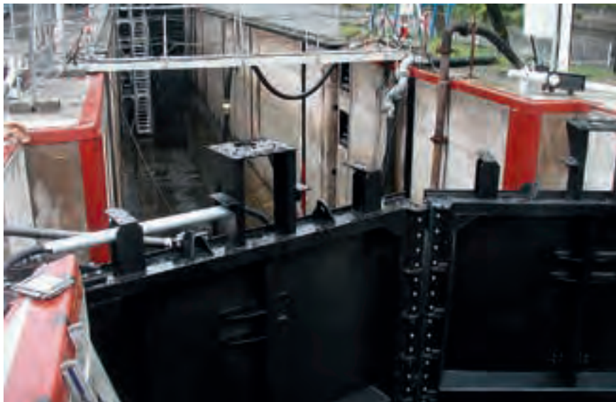
Figure 8.03: Mounting the closing elements avoiding constraint forces and leakage
