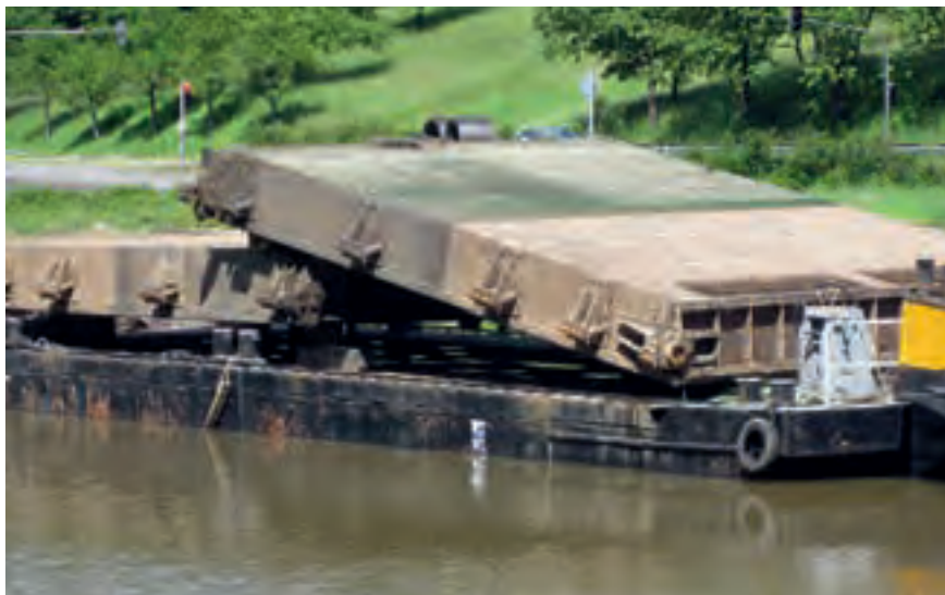
Figure 4.34: Large lock gates ready for overhaul
