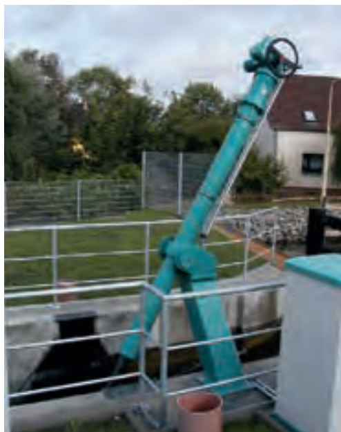
Figure 2.067: Handwheel/motor change-over only possible using tools
