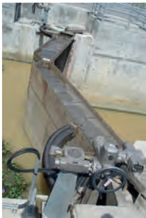
Figure 3.25: Mitre gates operated via rounded toothed racks
