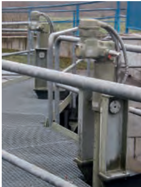
Figure 4.38 Actuators with red motor-manual operation change-over lever and square for power tool operation
