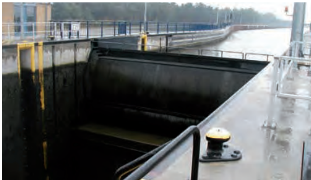
Figure 1.27: Radial gate with compression gate arms
