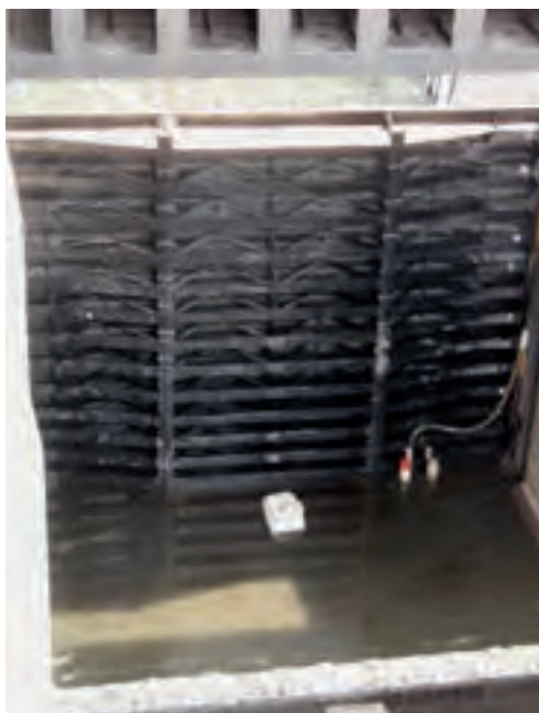
Figure 8.09: Stop log weir below the lift gate of a lock
