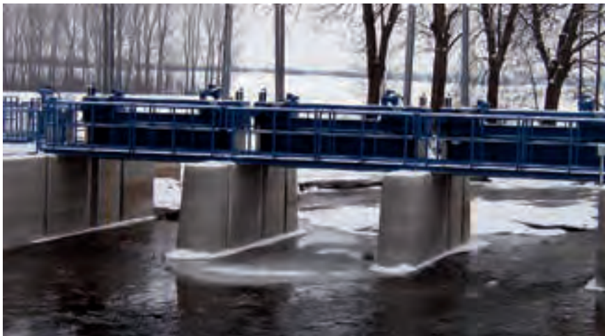
Figure 2.134: (N-1) rule: If a waterway cannot be opened, the remaining waterways ensure water drainage
