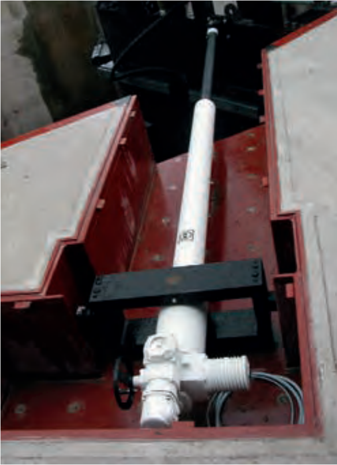
Figure 4.21: Actuator with lifting cylinder in basic sizes at mitre gate
