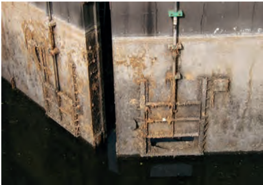
Figure 2.042: Strongly polluted and sluggish mitre gates
