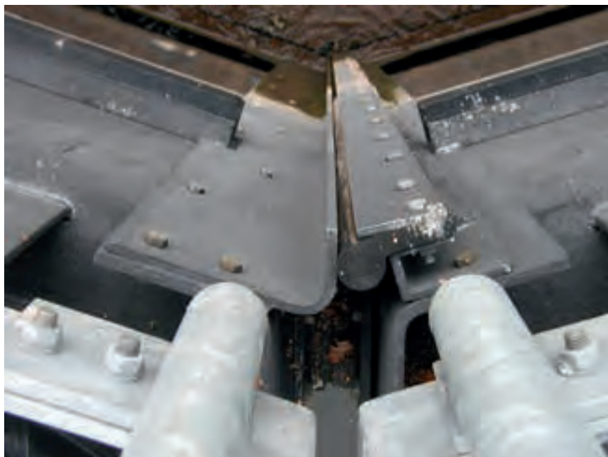
Figure 4.18: Bulb and tail seal at mitre gate
