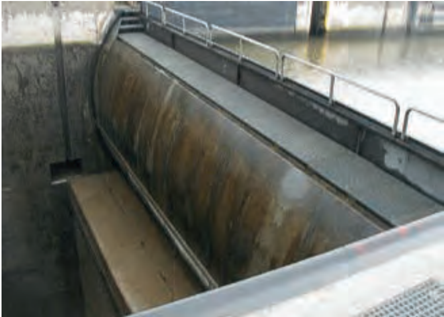
Figure 4.35: Radial gate with tension gate arms as upper lock gate
