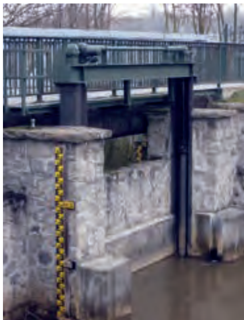
Figure 2.088: Spindles protected by tube at a sluice gate in front of a baffle (Elster 2 1 weir)
