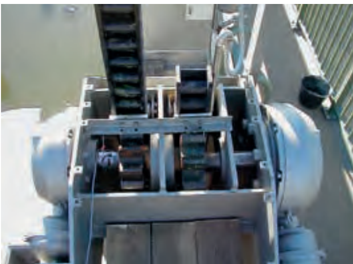
Figure 2.104: Pinion shafts in parallel to flow direction
