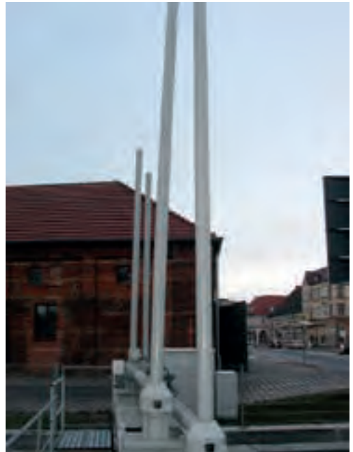
Figure 2.083: Bent stem protection tube
