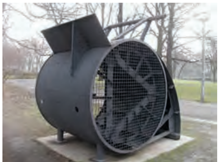
Figure 7.09: Roller gate weir with gate shield on top and gate shield with sealing strip at the bottom, cutout
