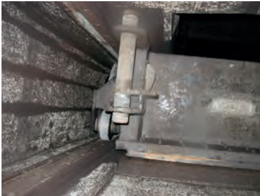
Figure 8.15: Locking bolt at a roller gate
