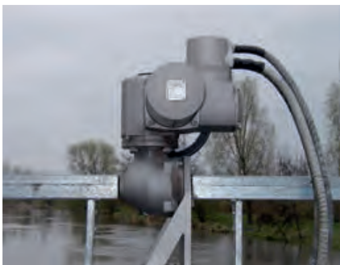
Figure 2.057: Bevel gearboxes with electric actuator, central mount
