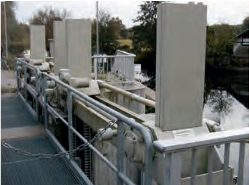
Figure 5.03: One cover protects respectively two lantern gears
