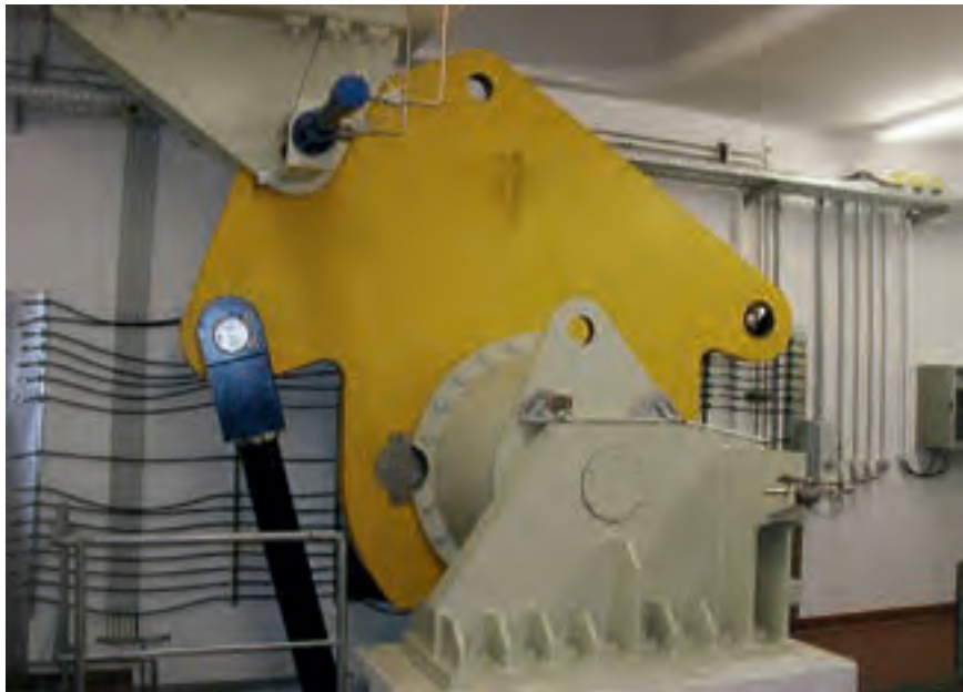
Figure 4.36: Pivot mounted radial gate with hydraulic cylinder in an underground service room below the lock
