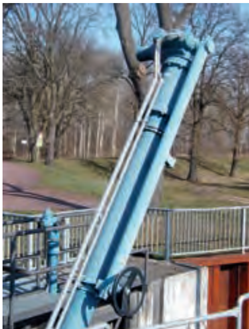
Figure 2.071: Manual operation with covered chain guide
