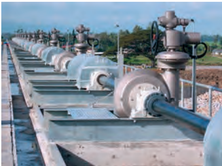
Figure 2.113: Actuator/gearbox combination between respectively two cable drums
