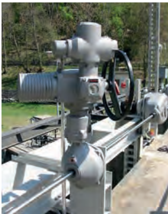
Figure 2.095: Anti-backdrive device between actuator and bevel gearbox
