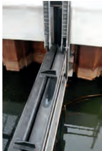
Figure 4.13: Cross-over protection at double sluice gate
