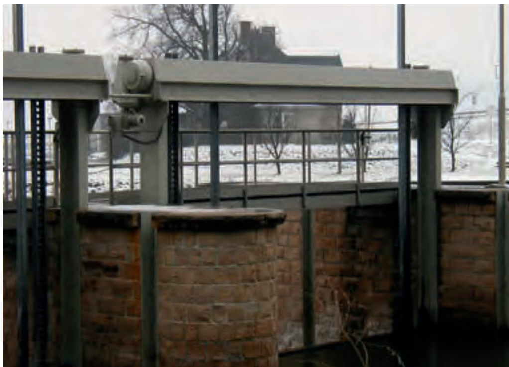
Figure 2.105: Side mount of actuator and worm gearbox for two pinions
