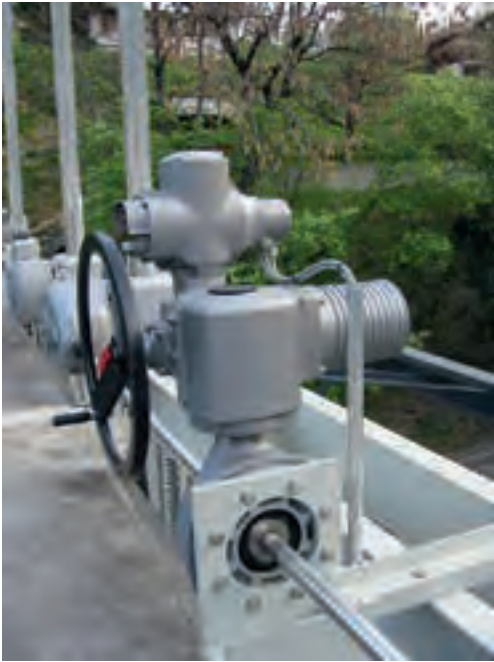
Figure 2.058: Bevel gearbox with through-shaft
