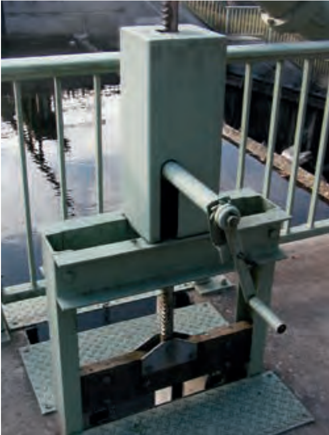
Figure 2.089: Toothed rack and pinion – enclosed – with crank handle
