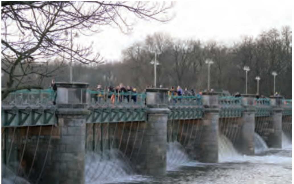
Figure 1.06: The weir is operated with hand winches
