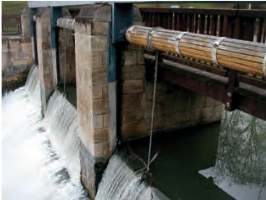
Figure 7.04: Sluice gate weir with ancient chain hoist and modern rack and pinion hoist
