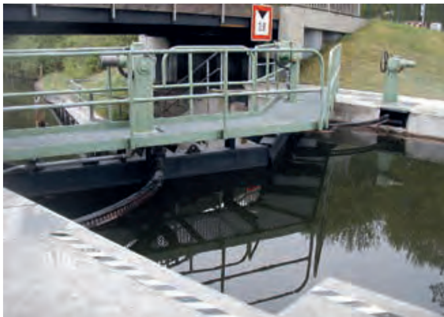
Figure 3.24: Lantern gear segments at a mitre gate
