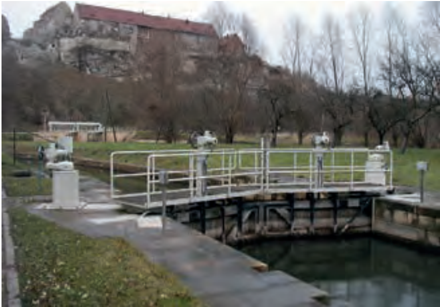
Figure 7.02 Wooden mitre gate in sandstone chamber, original condition was restored
