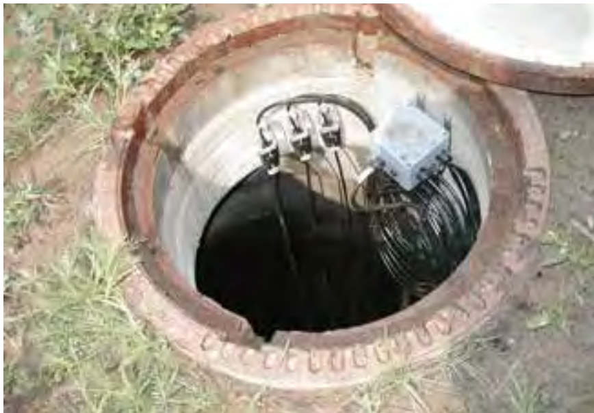
Figure 4.14: Measurement point installation in a pit
