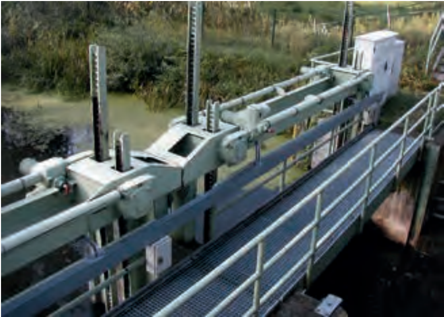
Figure 2.128: The handwheels and their extensions were dismantled and stored
