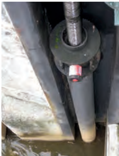
Figure 2.087: Spindle nut on a protection tube
