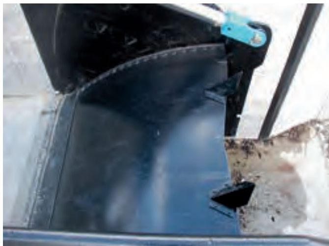
Figure 2.142: Fish-belly flap gate with flow deflector and V-notch
