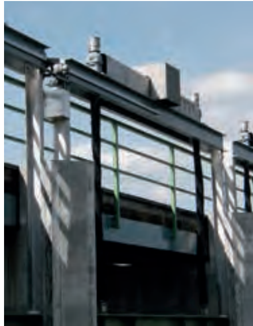
Figure 2.086: Lowered spindle with retracted spiral protection and extended bellows
