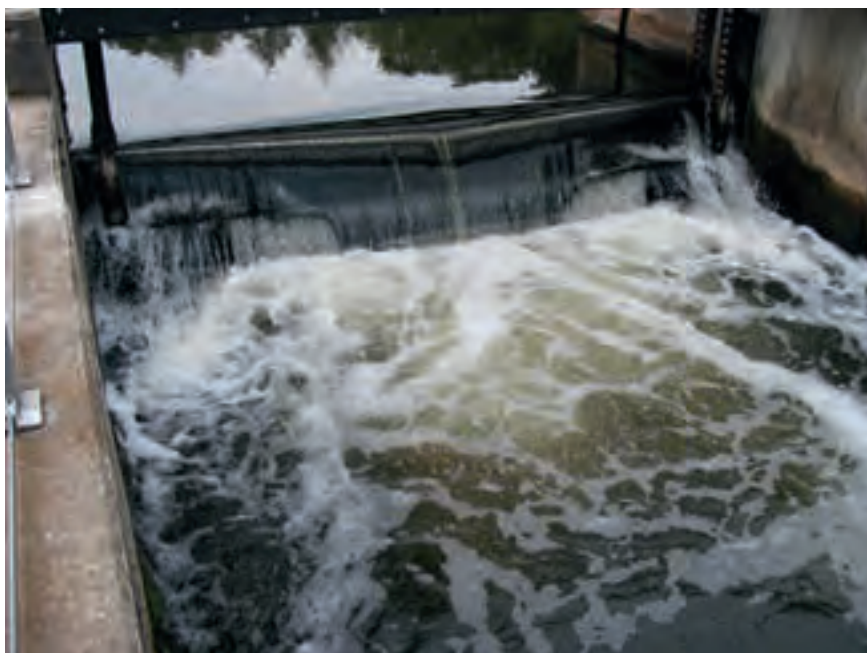
Figure 2.125: Upper gate with V-notch
