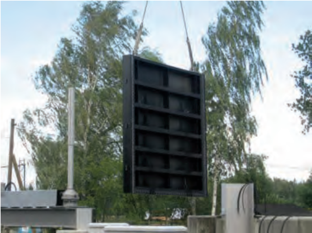
Figure 2.012: Tailwater side of a sluice gate with bars, slide and sealing strips
