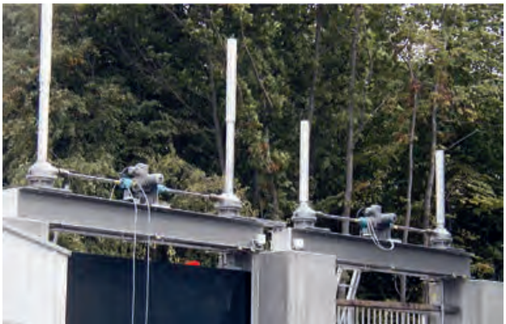
Figure 2.084: Telescopic protection tubes in Open and Closed positions of sluice gate weirs
