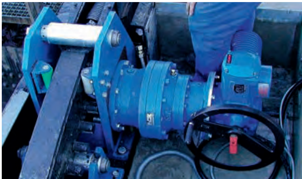
Figure 3.28: Buckled lantern gear with pinion, planetary gearing and actuator for a flap gate
