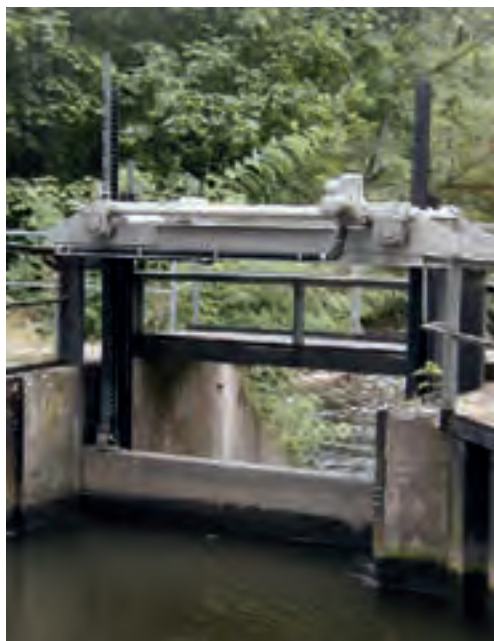
Figure 2.102: One actuator operates two worm gearboxes
