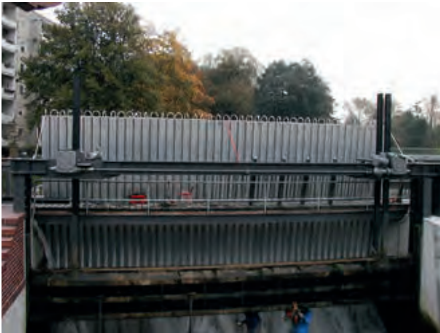
Figure 8.10: Blocking a shutter weir by a needle weir consisting of metal pipes
