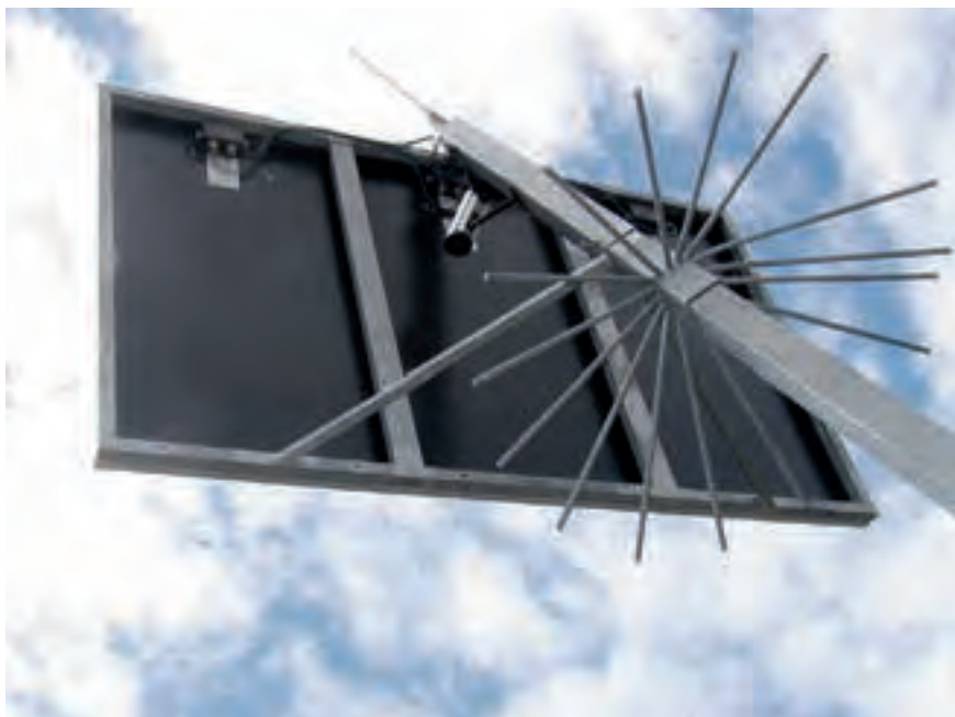
Figure 4.23: Solar module with supervision camera and anti-climb guard
