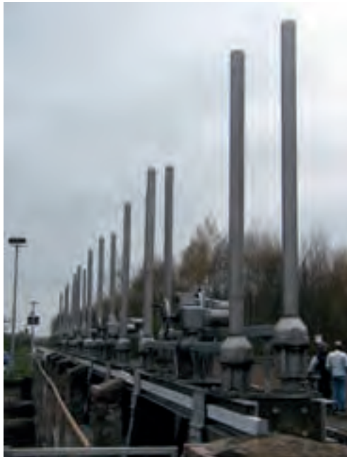
Figure 2.082: Compact stem protection tubes mounted on bevel gearboxes
