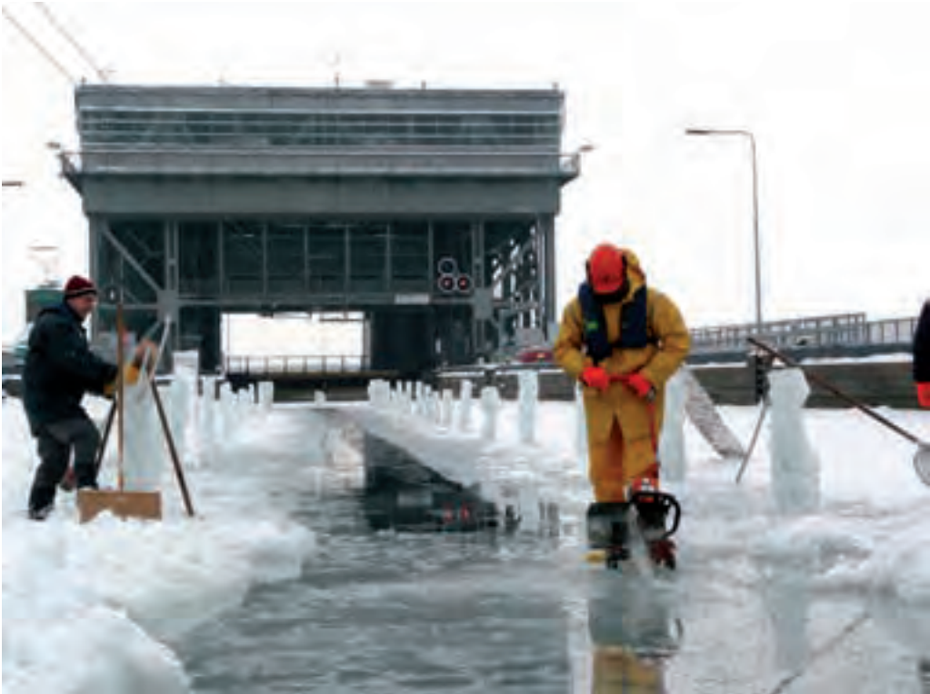
Figure 2.031: A longitudinal cut into the ice brings relief for the ship lift at Niederfinow and the subsequent canal bridge. One man acts as security officer.
