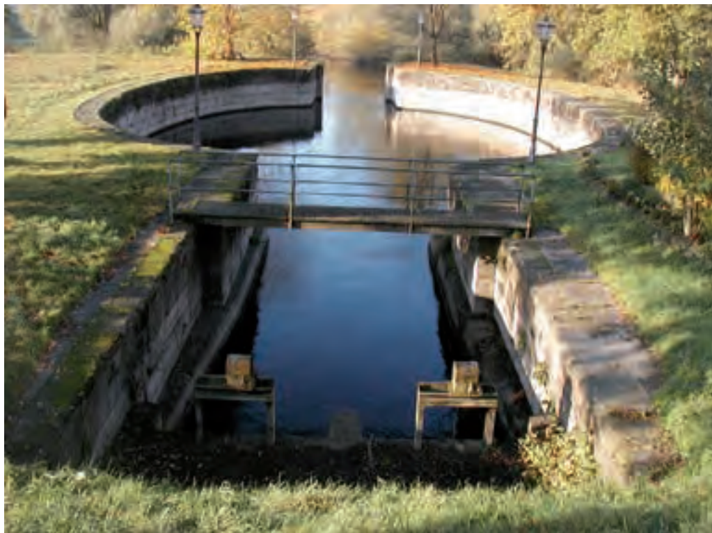
Figure 1.23: Old foursquare lock
