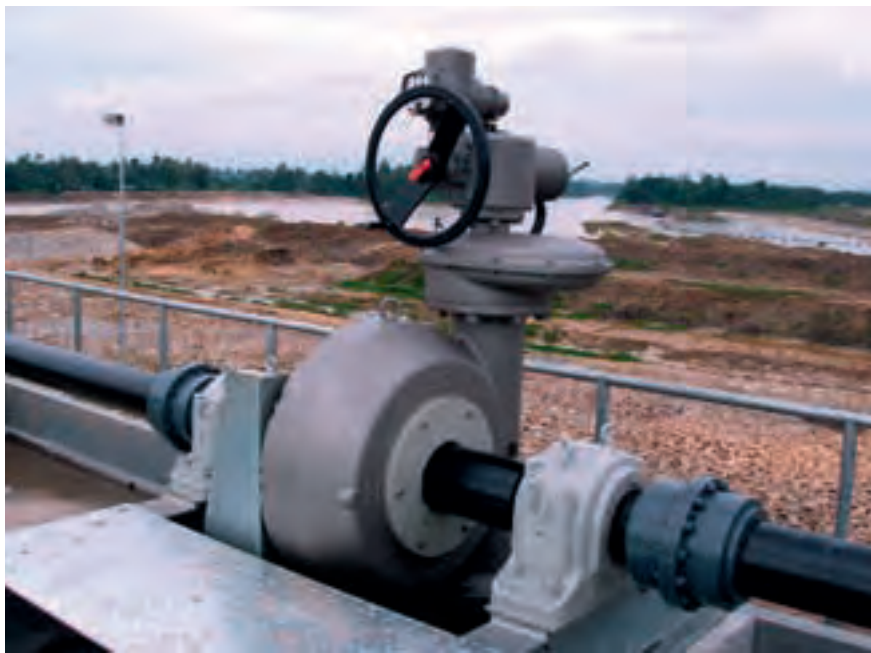
Figure 2.114: AUMA MATIC actuator controls mounted on an actuator/gearbox combination
