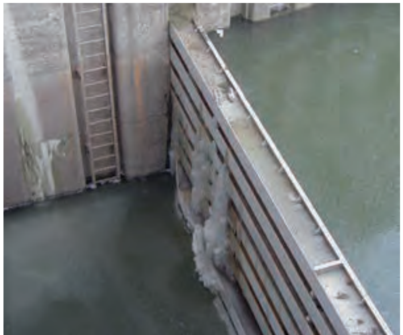
Figure 2.030: Impact ice force onto an inspection gate from both sides at different heights
