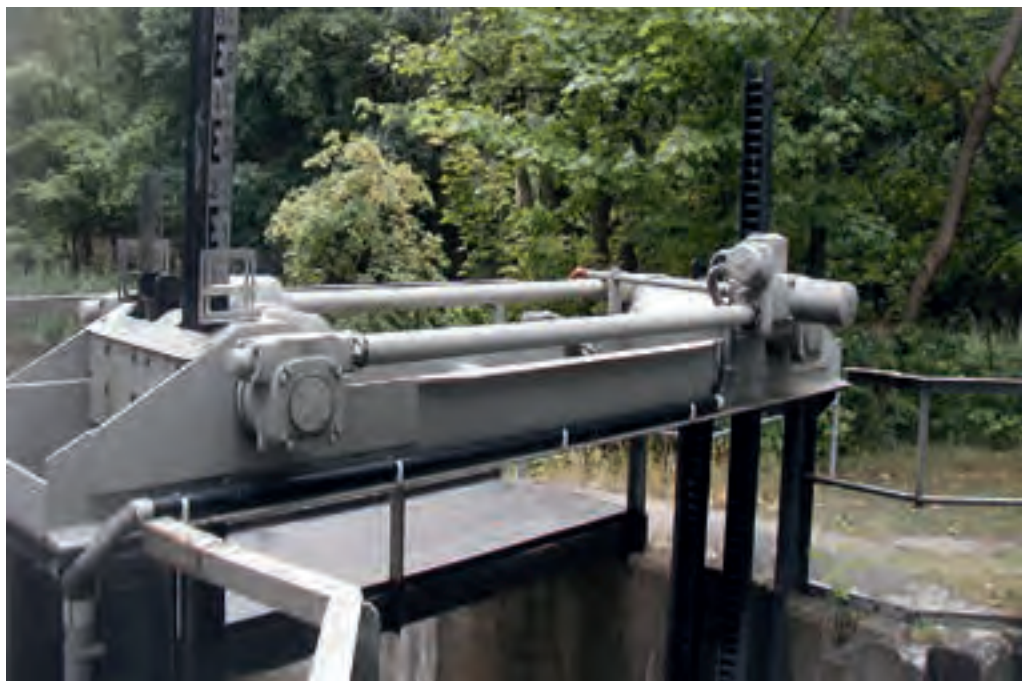
Figure 9.02: New: Enclosed worm gearboxes and actuators for motor operation
