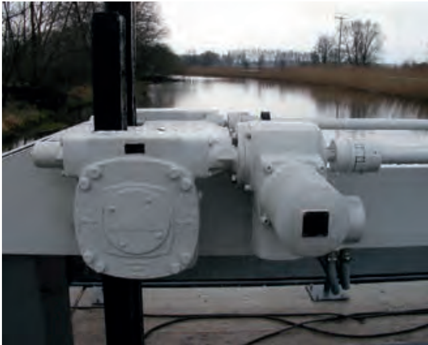
Figure 2.092: Worm gearbox with actuator
