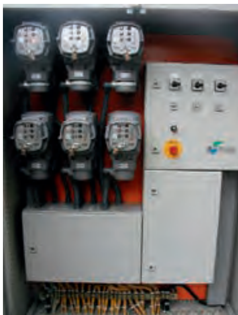
Figure 6.05: AUMA Matic actuator controls on wall brackets in a lockable control cabinet
