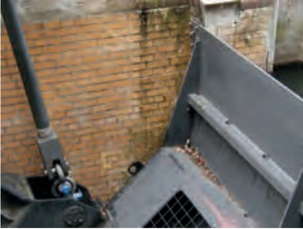
Figure 8.13: Two mounting lugs – lower centre of the picture and counterpart – allow mechanical locking of the segment gate
