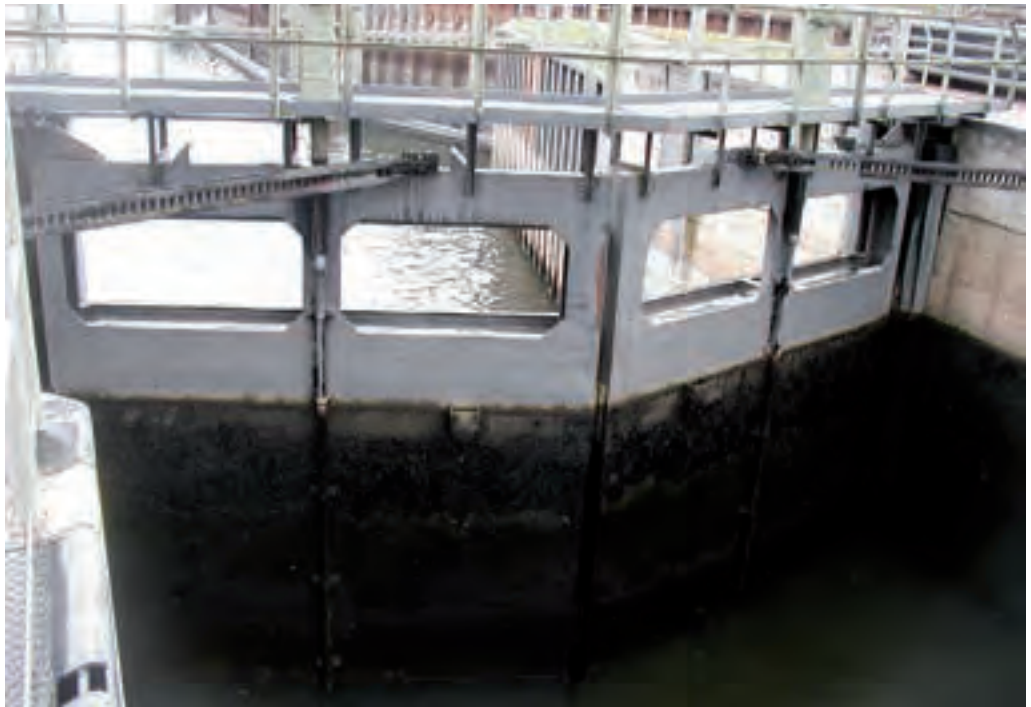
Figure 2.032: Lower lock gates with drains for ice and flood drainage
