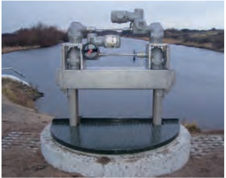
Figure 5.04: Actuator technology of a double sluice gate with open and accessible shafts
