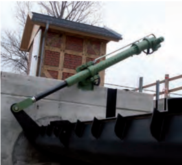
Figure 1.15: Fish-belly flap weir
