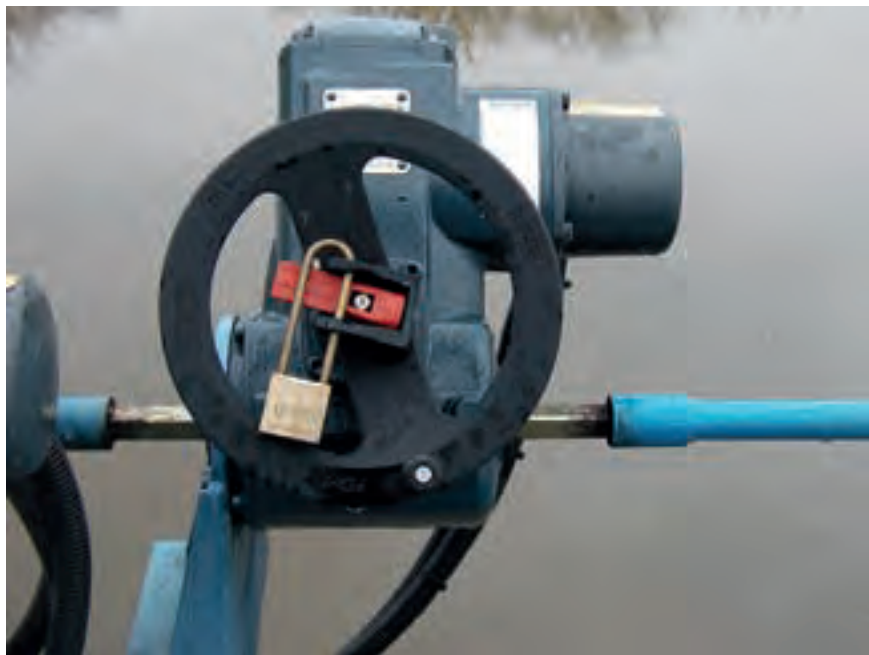
Figure 6.01: Lockable handwheel
