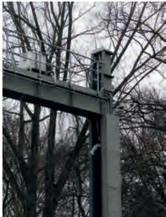
Figure 8.14: Lockable hook (lower centre of the picture) to maintain a lock lift gate
