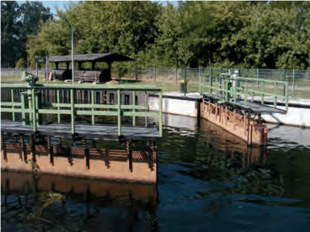
Figure 3.26: Improvement by self-locking actuators: slowed-down gate operation of a mitre gate lock
