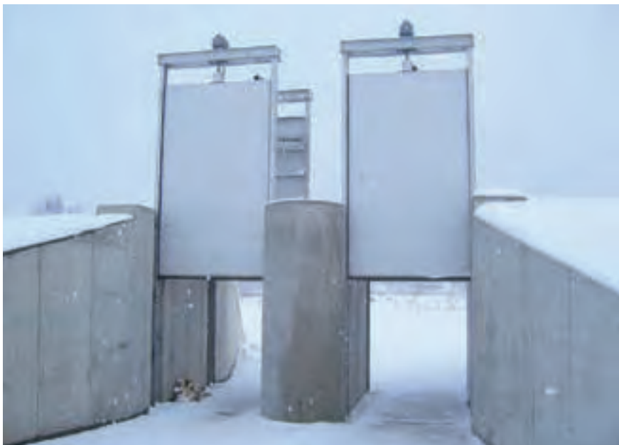
Figure 2.002: Sluice gates weirs with one connecting element
