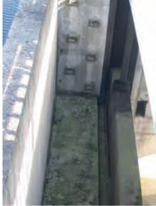
Figure 2.006: View from the top onto a flood protection sluice gate: from left baffle – head block – head seal – sluice gate
