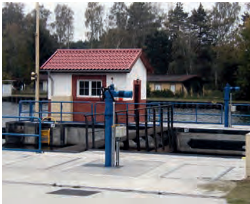
Figure 2.093: Actuators with brake motors at lock by-passes
