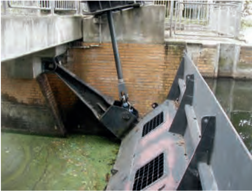
Figure 2.144: Compression gate weir in Berlin Spandau with electrical lifting cylinder
