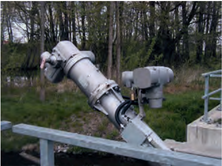
Figure 6.03: Lockable protection cover at AUMATIC local controls
