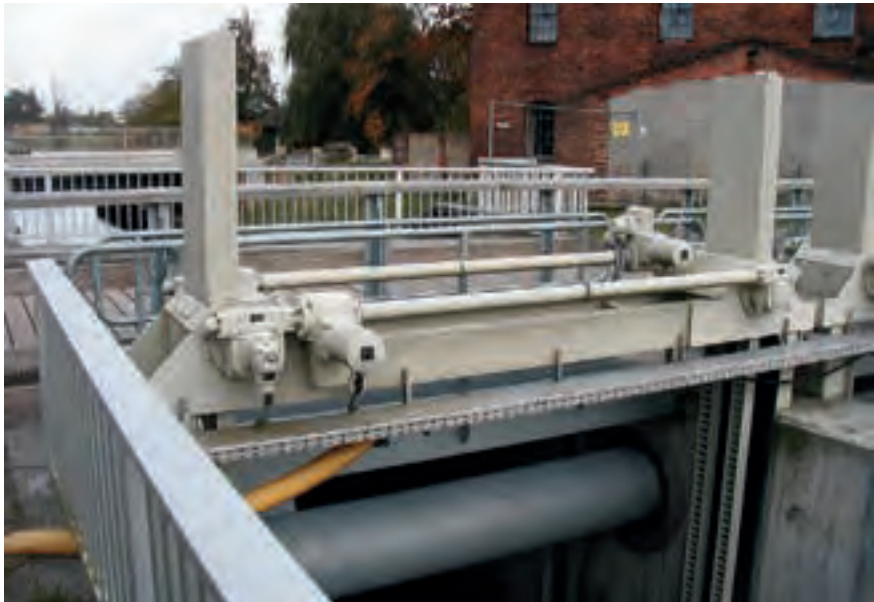
Figure 4.10: Position indicator at output drive to pinion of lantern gear
