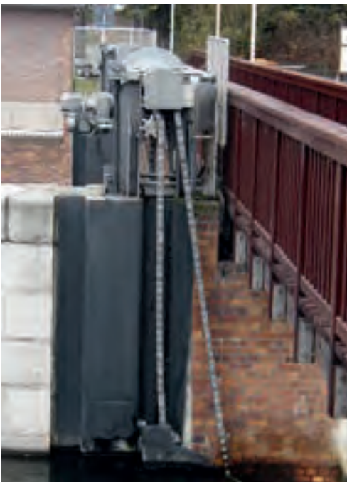
Figure 2.154: Sluice gate and shutter movement are made by a joint chain
