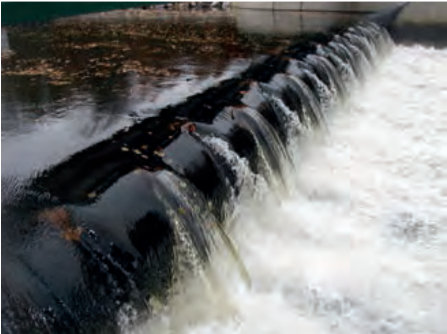
Figure 4.05: Inflatable weir with flow deflectors
