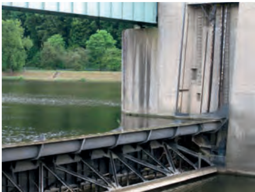
Figure 2.155: Combined weir subject to undercurrent
