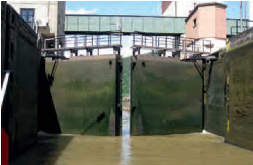
Figure 4.33: Large lock with hydraulic cylinders
