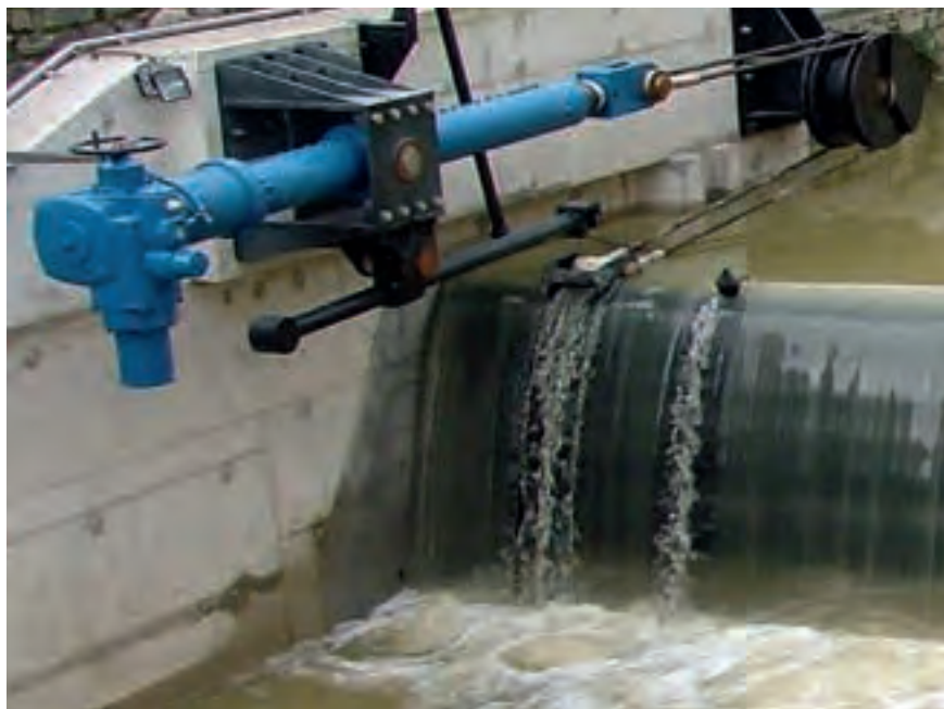
Figure 2.149: Flap actuating gear with pulley
