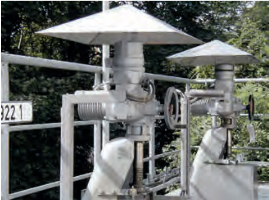
Figure 4.19: Sun shades mounted on actuators
