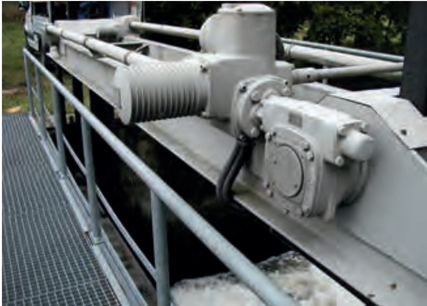
Figure 2.107: Worm gearbox pair: RR at actuator output and LR at the opposite side with shaft located above
