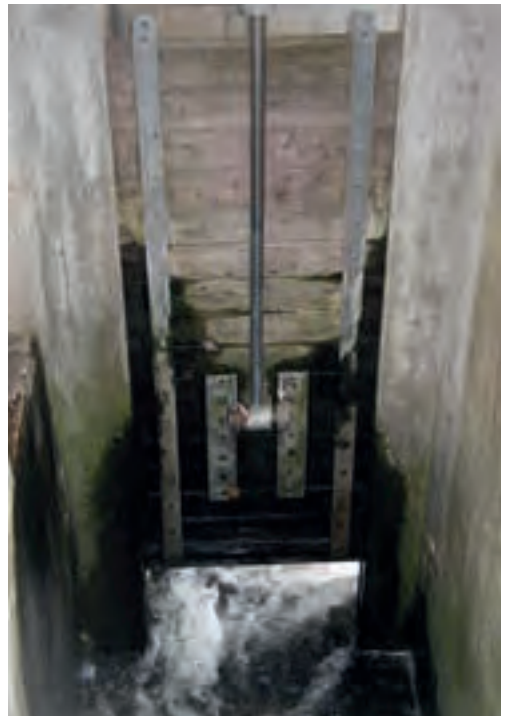
Figure 4.26: Hydraulically operated sluice gate
