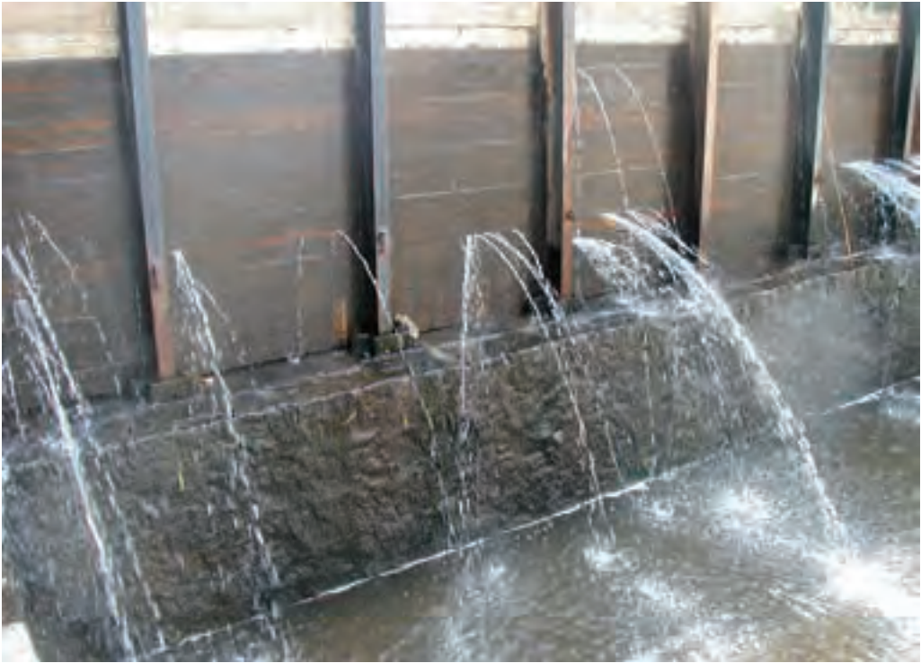
Figure 1.02: Stop log weir
