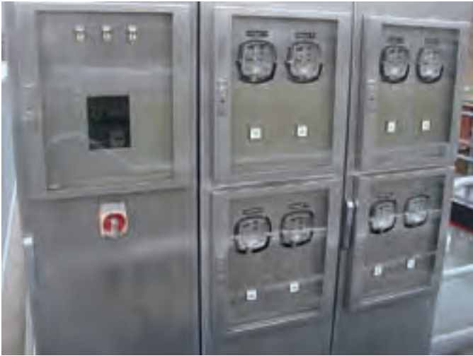
Figure 6.06: AUMA MATIC local controls behind lockable glass doors
