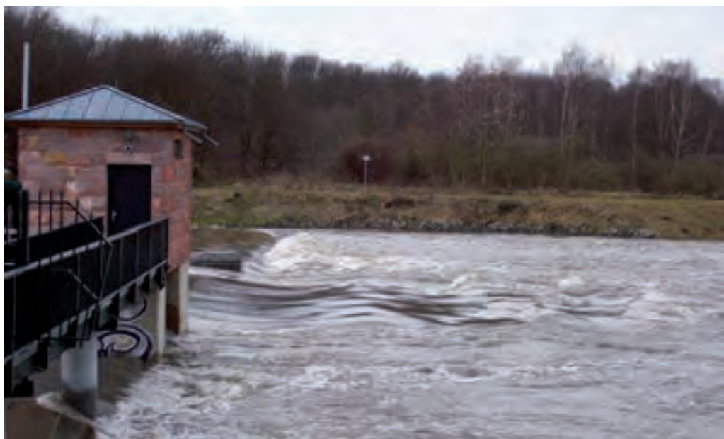
Figure 1.21: Same installation as figure 1.20: the flood water drains below or above opened locks and a fixed weir.
