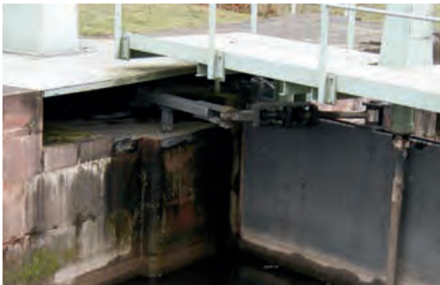
Figure 3.22: Toggle lever at a mitre gate led via pinions
