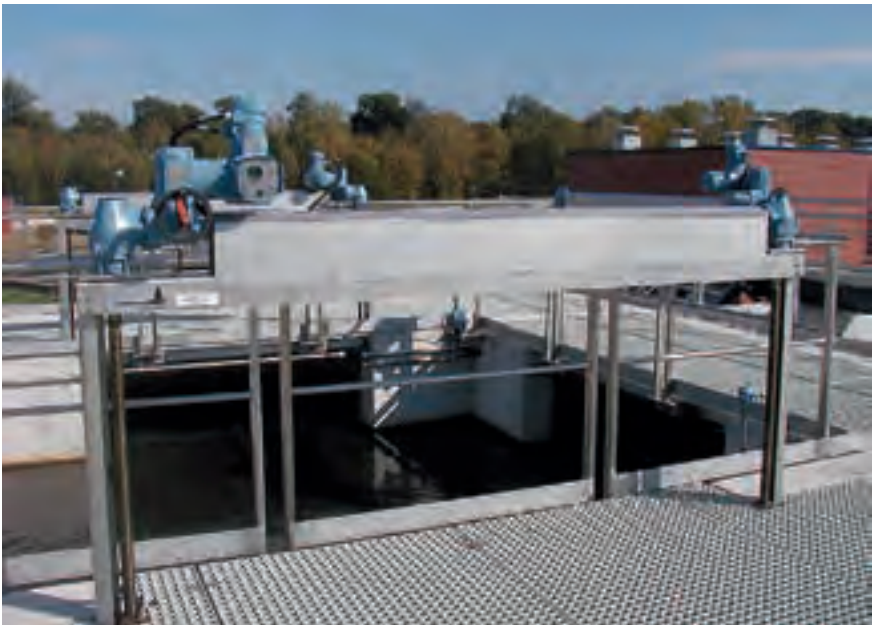
Figure 4.08: Actuators with AUMATIC (AC) actuator controls on a double-stem gate valve
