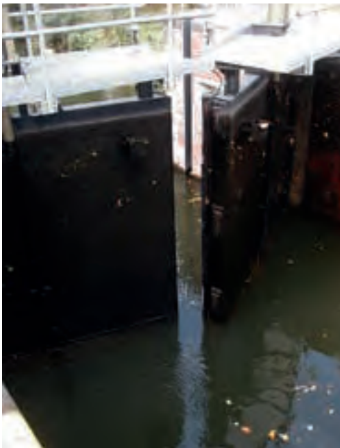
Figure 4.17: Uneven closing of mitre gates
