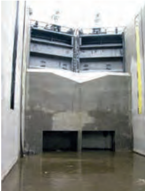
Figure 3.07: Headwater gate: Smooth water inflow via the inlets located in the chamber floor
