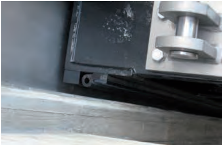
Figure 2.019: Sluice gate with suspension, slide strip and sealing strip in bulb and tail profile
