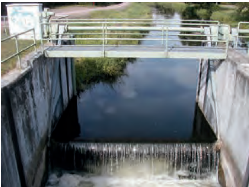
Figure 2.147: Shutter with two-sided cable winch and one worm gearbox
