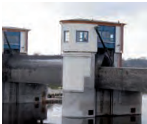
Figure 1.16: Combined weir: Sluice gate with vertical (left) and horizontal (right) flap gate
