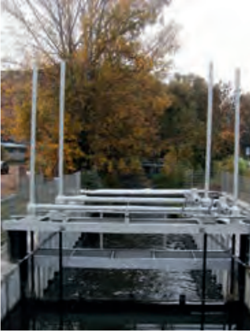
Figure 2.121: Double sluice gate with spindle actuators mounted one behind the other
