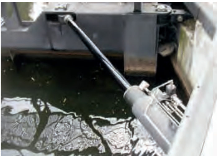
Figure 4.32: Mitre gate with hydraulic cylinder for gate operation
