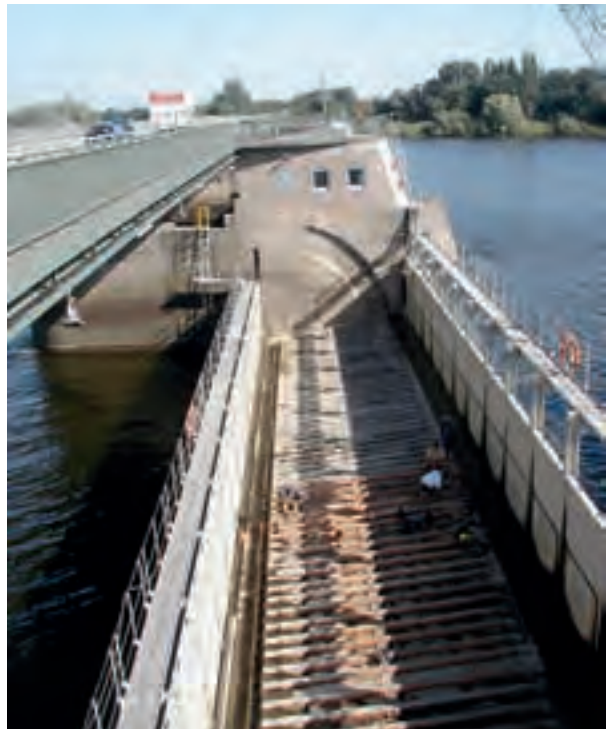
Figure 8.12: Laterally placed inspection gates protect a sector weir
