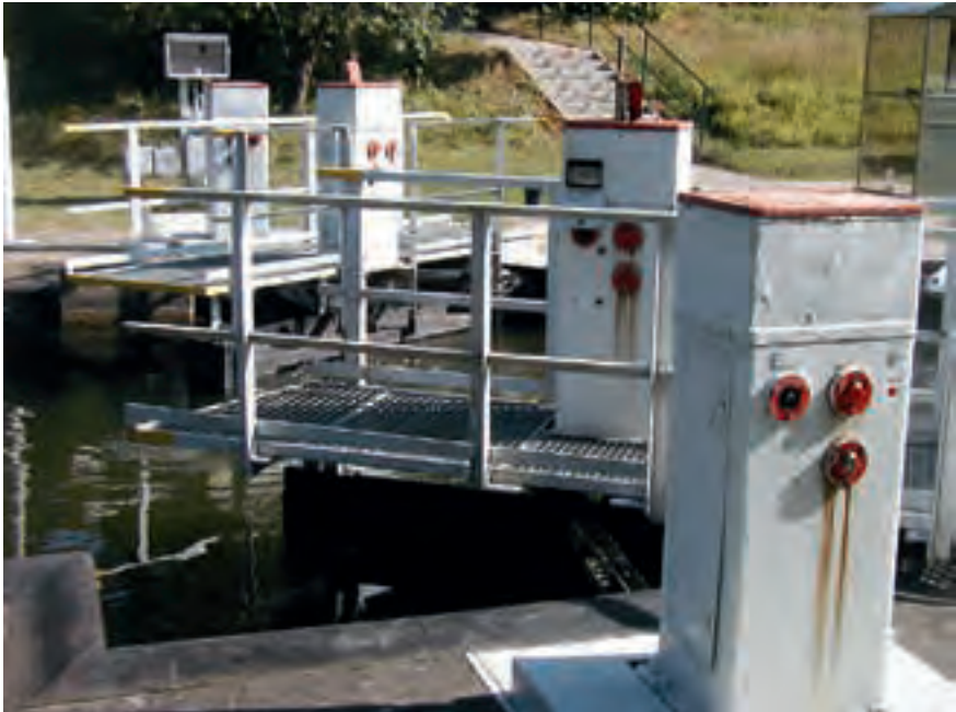
Figure 9.08: Former: Mitre gate lock with enclosed actuators and gearboxes
