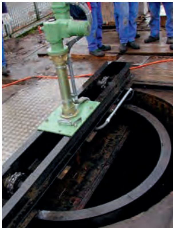
Figure 3.14: Cylindrical gate with actuator and linear thrust unit at the by-pass of a lock gate
