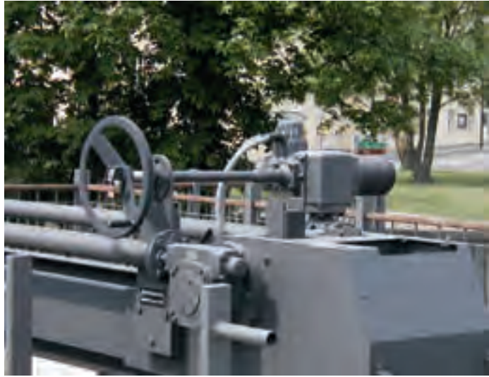
Figure 2.069: Actuator with handwheel spindle extension
