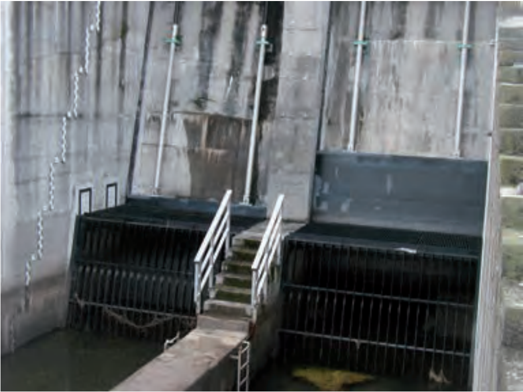
Figure 2.021: In this case, tilting of sluice gates achieves an increase in buoyant force when opening for rear inflow
