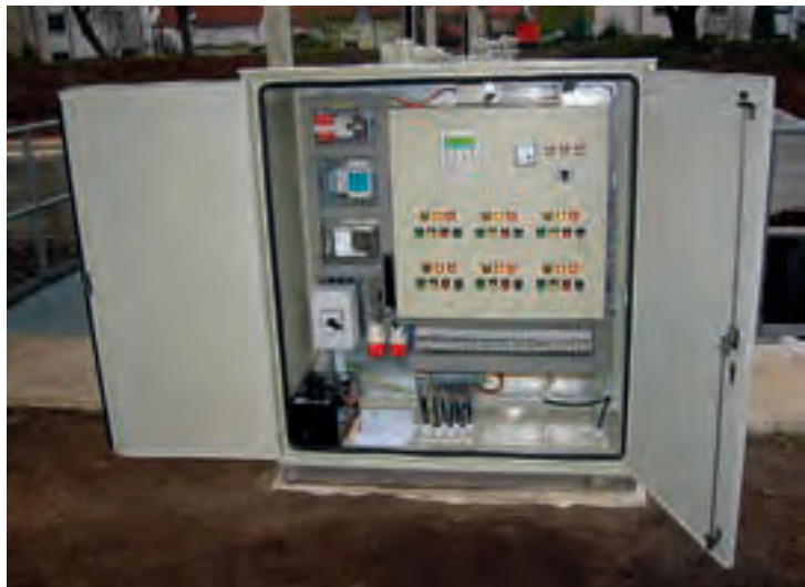
Figure 4.44: Control cabinet with voltage supply via generator
