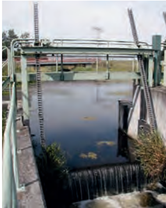
Figure 2.145: Shutter operated manually via primary reduction gearing; pinions engage into lantern gears without additional gearboxes
