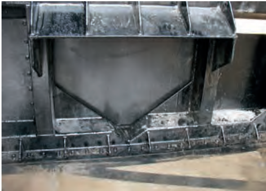
Figure 4.16: Roof of a sluice gate for settling the water surface
