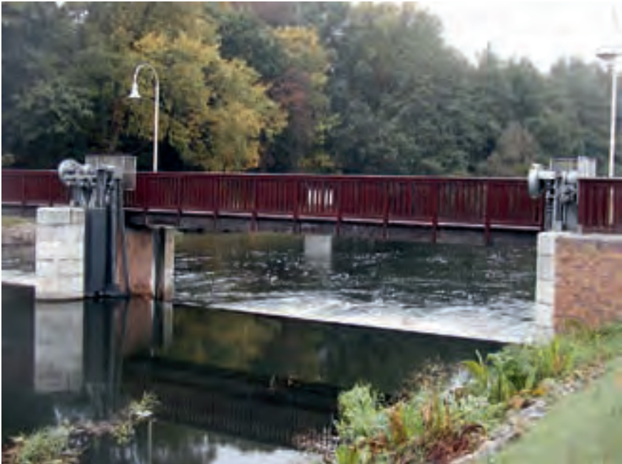
Figure 2.153: Sluice gate weir with fine regulation via flap gate. Both sides are driven by one actuator respectively
