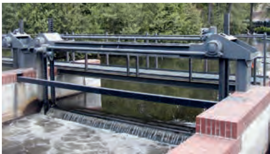
Figure 2.131: Worm gearbox pair: RR at the actuator output, left in the picture, and LR right
