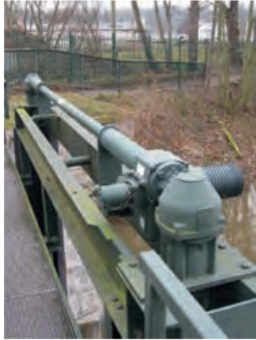
Figure 2.059: Bevel gearboxes with electric actuator, side mount
