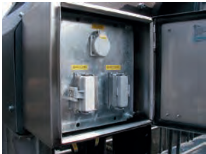
Figure 6.07: Service entries for two weir segments
