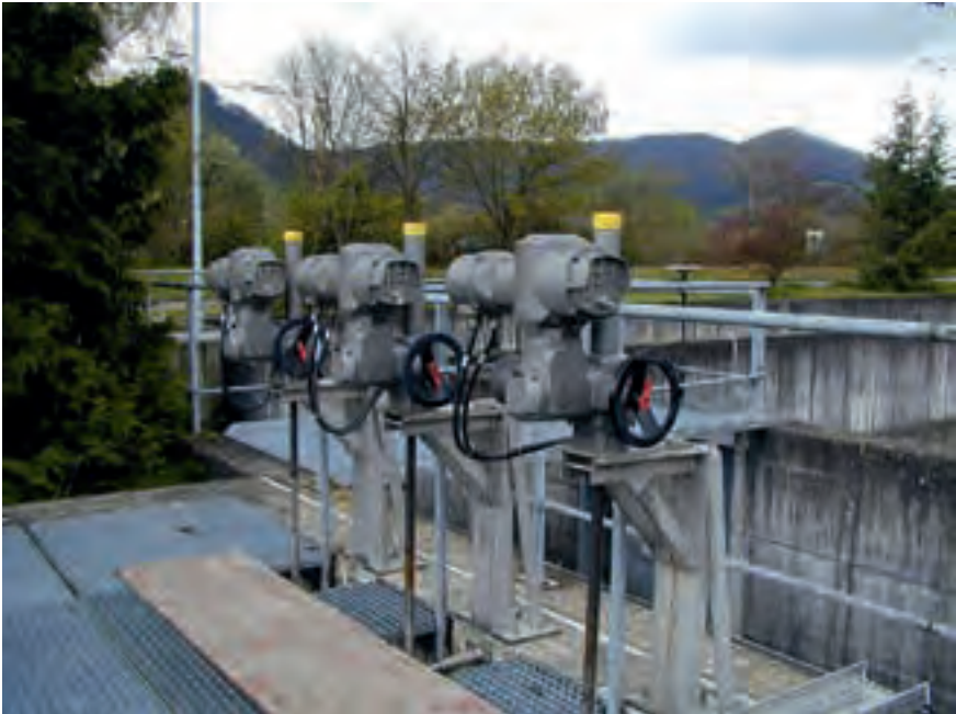
Figure 4.07: Actuators with AUMA MATIC (AM) actuator controls on single-stem gate valves
