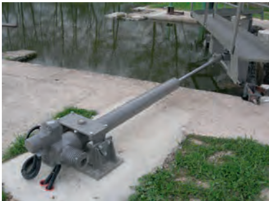
Figure 3.20: Mitre gate operation via electrical lifting cylinders
