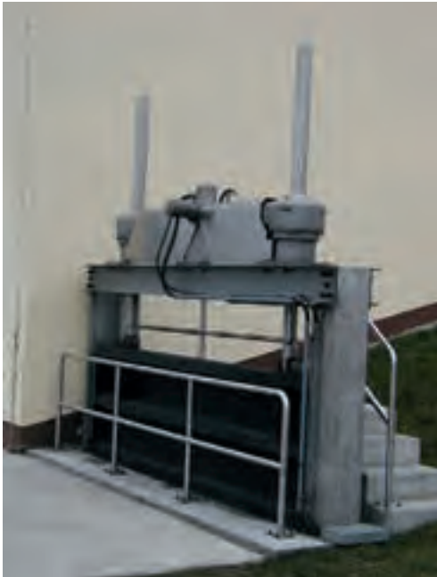
Figure 2.054: Actuator and 2 bevel gearboxes with adjustable output direction of rotation
