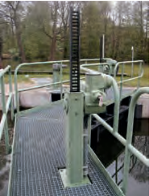
Figure 3.13: Lantern gear gate mechanism at a mitre gate
