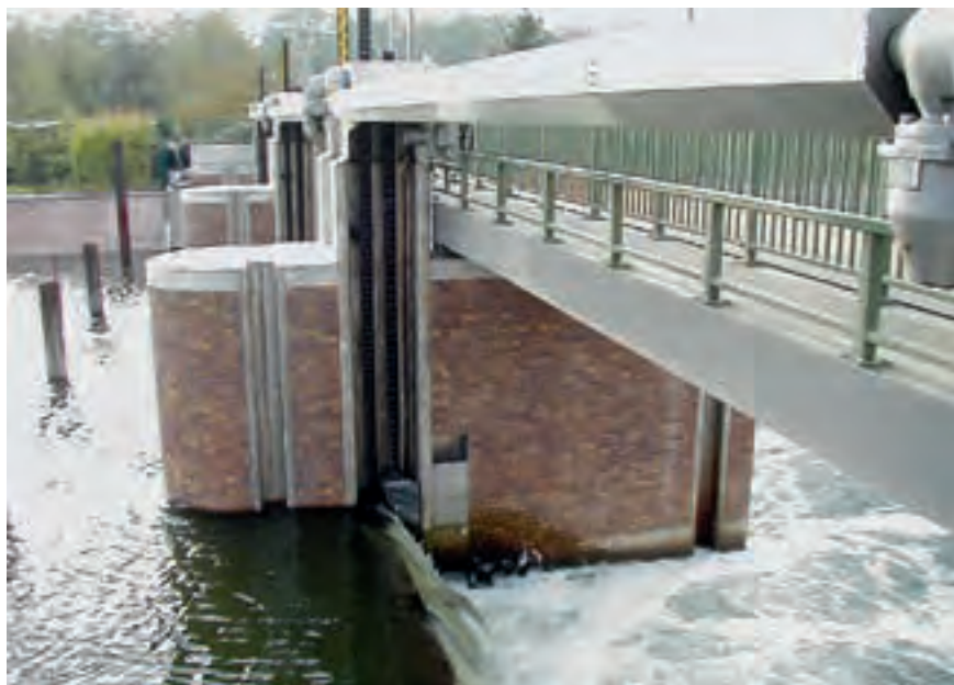
Figure 2.123: Double sluice gate with lantern gears in a pier recess
