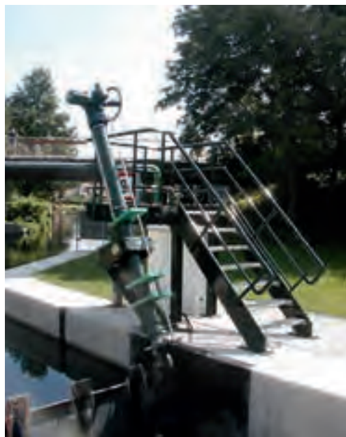
Figure 2.068: A stairwell for handwheel operation and maintenance
