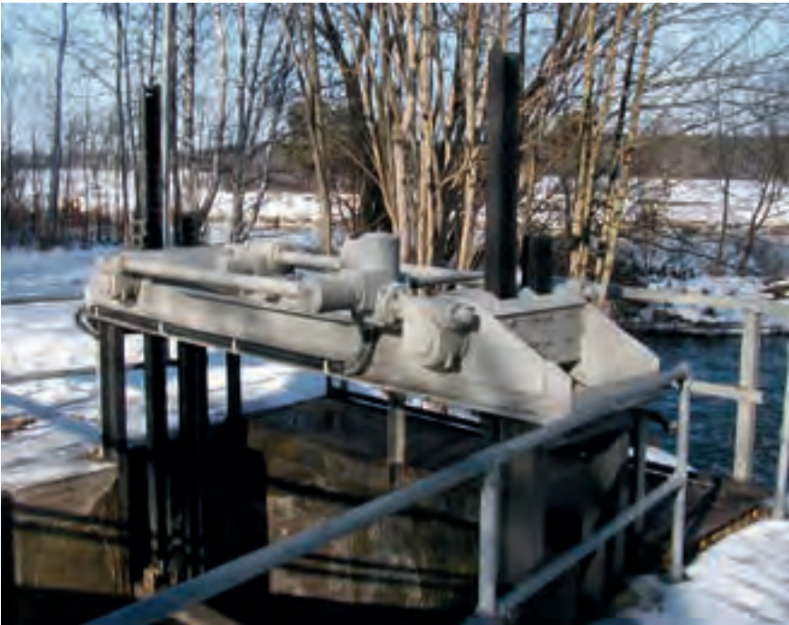
Figure 2.122: Double sluice gate with lantern gear drive mounted diagonally to each other
