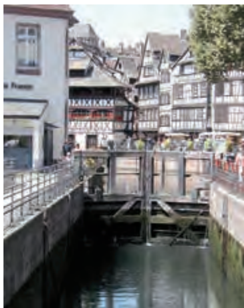
Figure 1.24: Mitre gate within upper gate
