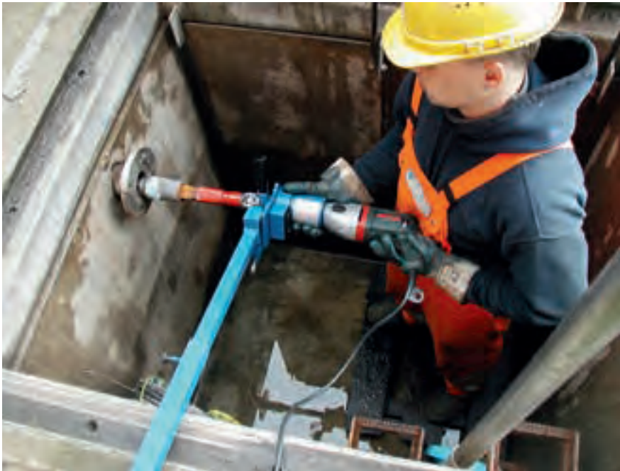
Figure 4.37: Drilling machine with distortion lock
