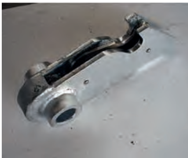
Figure 2.127: Latch or pinion hooks of water saving double gate
