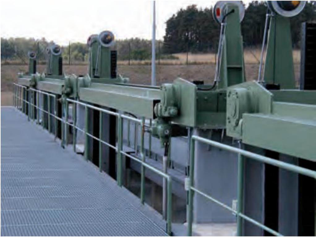
Figure 2.028: Sluice gate weir with cable drums for cables of slide and sealing rail heaters
