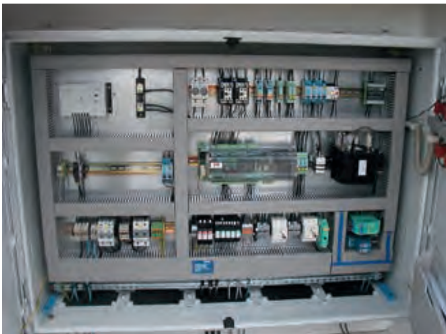
Figure 4.24: Site with solar controllers and modem
