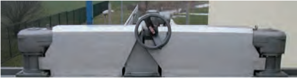
Figure 2.009: Actuator/gearbox combination option for a submerged gate
