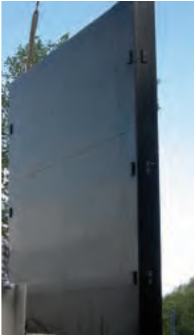
Figure 2.018: Sluice gate with guide blocks
