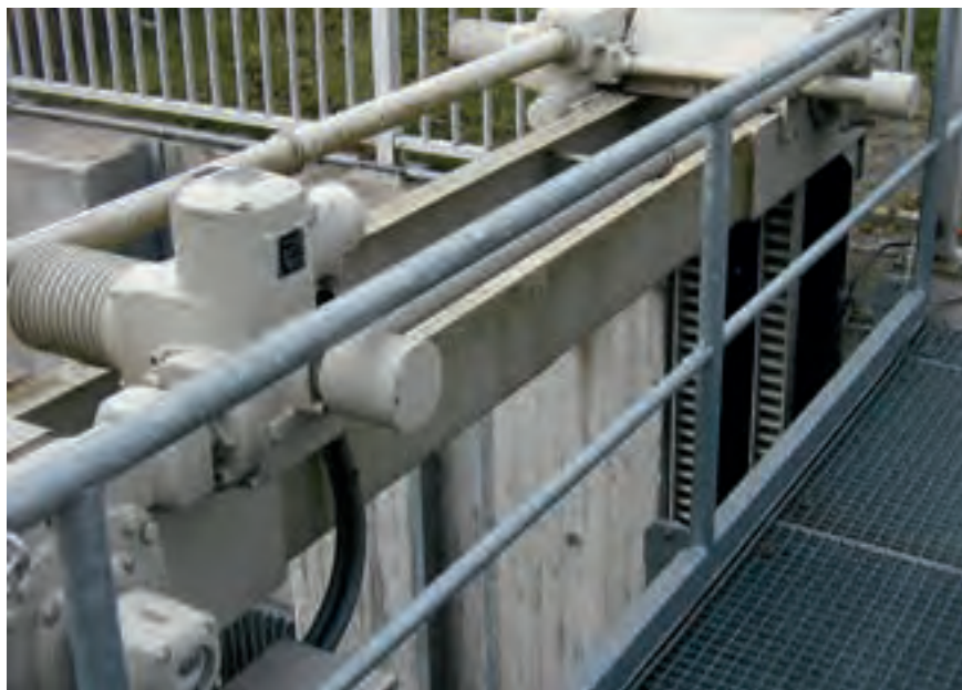
Figure 2.130: Upper and lower gate operation from one side. Lever arrangements and handwheel connection are enclosed
