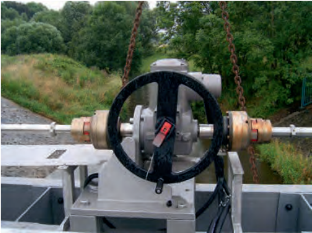
Figure 2.065: Elastic safety couplings with torque monitoring at an actuator
