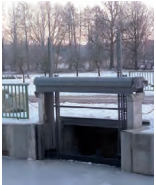
Figure 2.029: Ice force applied onto a weir
