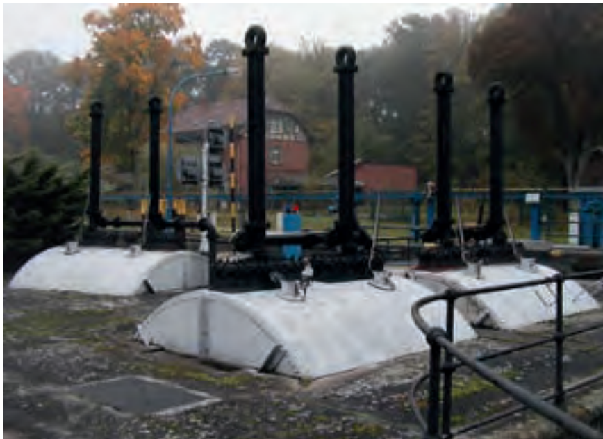
Figure 4.04: Hotopp siphon on a side basin of a lock for draining and filling the locks on both sides
