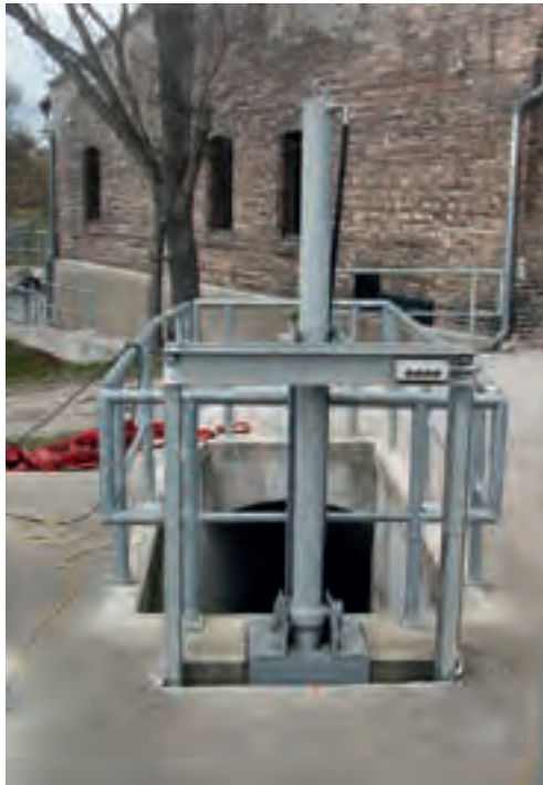
Figure 4.25: Hydraulic cylinder with local controls
