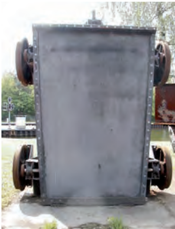
Figure 2.011: Wedge roller gate with running wheels and wheel flanges
