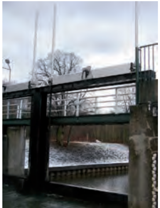
Figure 2.003: Sluice gate weir with two spindles
