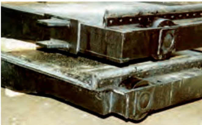
Figure 2.010: Roller gates, top: Upper side with lifting eyes and rubber sealing strip, bottom: Lower part with gasket and rubber sealing strip
