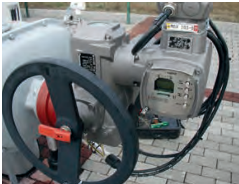
Figure 6.04: AUMATIC local controls without selector switch
