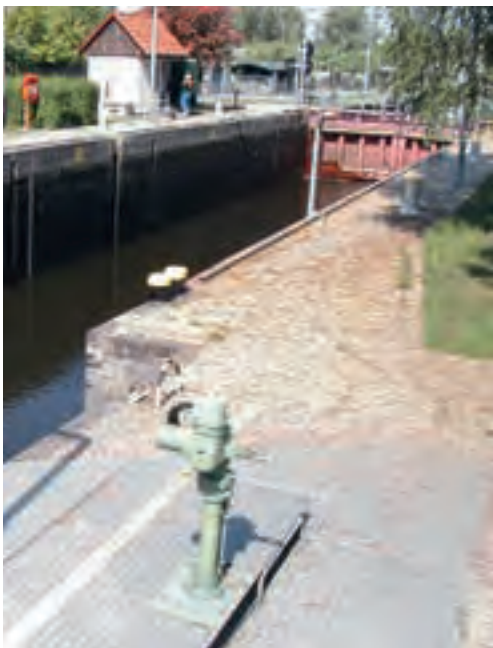
Figure 3.16: Lock chamber with by-passes. In front, the cylindrical gate drive of a by-pass. Opposite at the chamber wall: water inlet points marked in yellow
