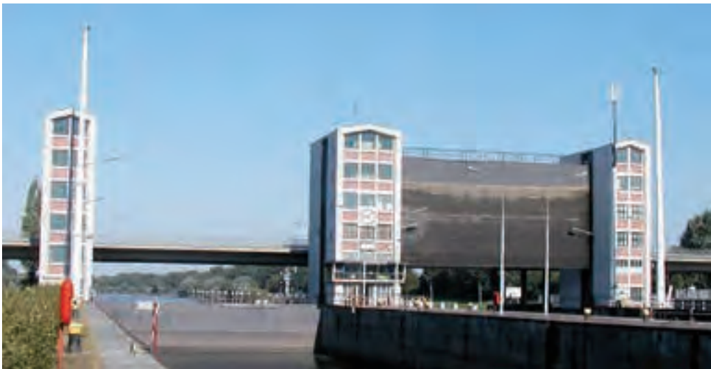
Figure 1.26: Open and closed lift gates
