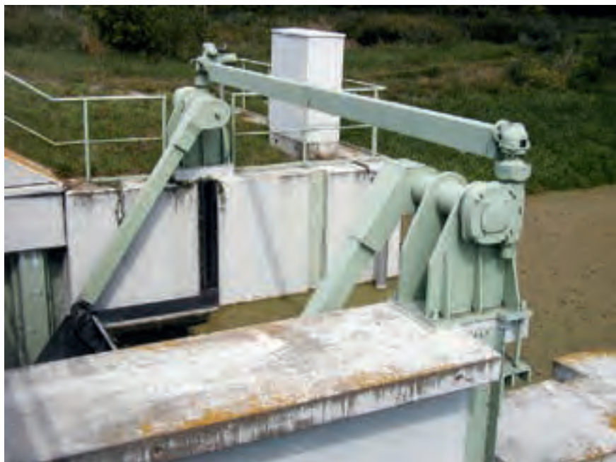
Figure 2.148: Shutter with two-sided cable winch and two worm gearboxes
