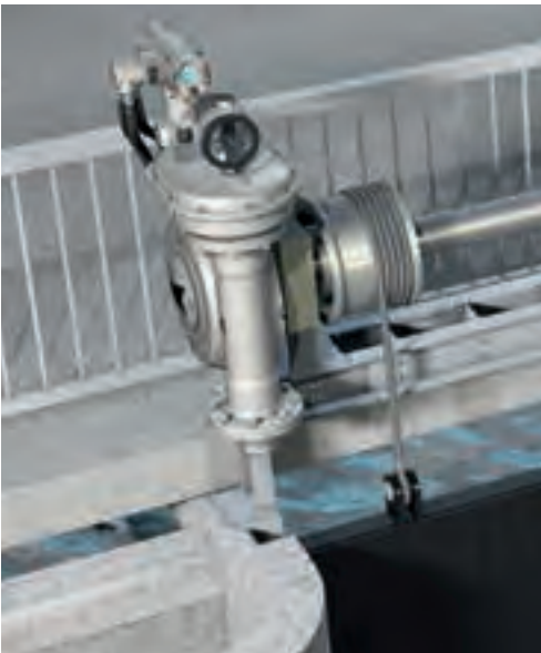
Figure 2.111: Actuator/gearbox combination with cable winch
