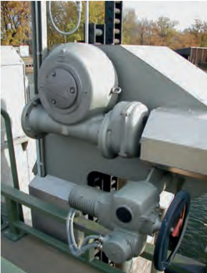
Figure 2.132: Actuator with connecting shaft for gearbox on head- water side (below)
