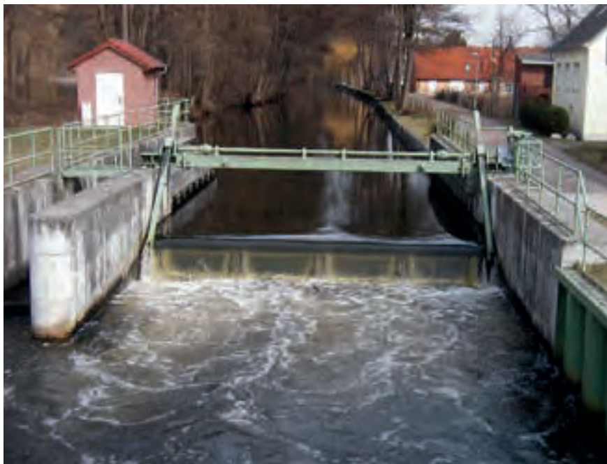
Figure 2.146: Shutter with two lantern gears and outside actuator with gearbox
