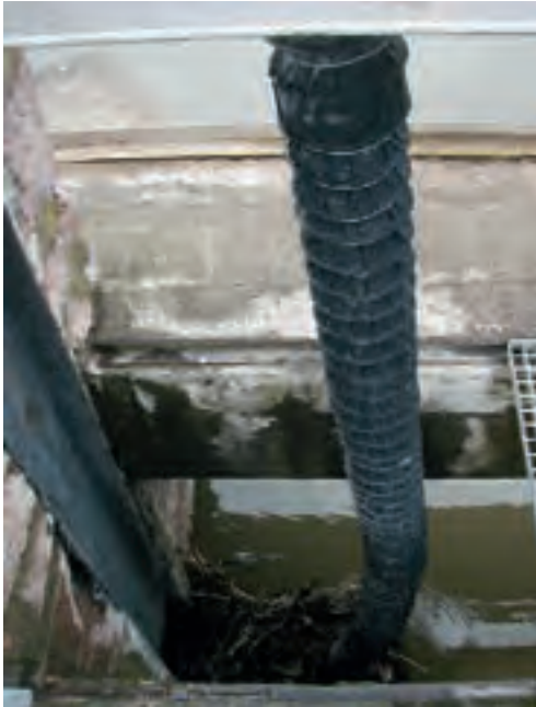
Figure 2.060: Buckled spindle
