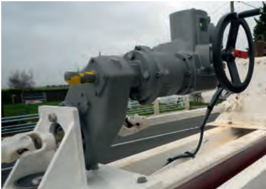
Figure 2.109: Centre mount actuator/anti-backdrive device/spur gearbox for pinion-lantern gear operation
