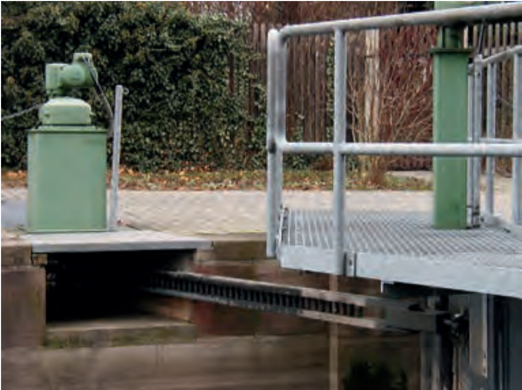
Figure 3.19: Mitre gate operation via lantern gear and pinion
