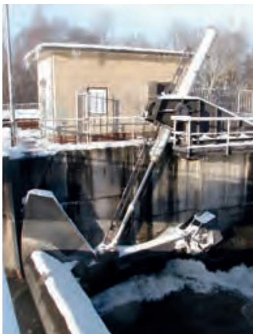
Figure 4.30: Hydraulic cylinder at a compression gate weir
